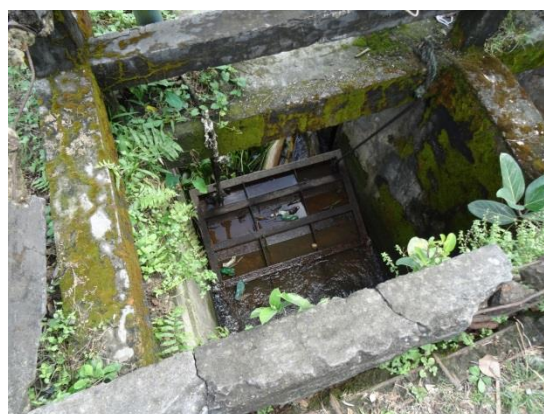
Picture 3.2: Bauria drainage sluice
