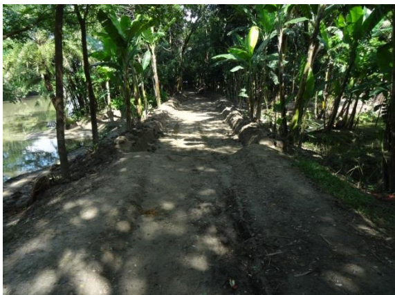
Picture 3.5: Elevated road next to khal in Gol Buaria area
