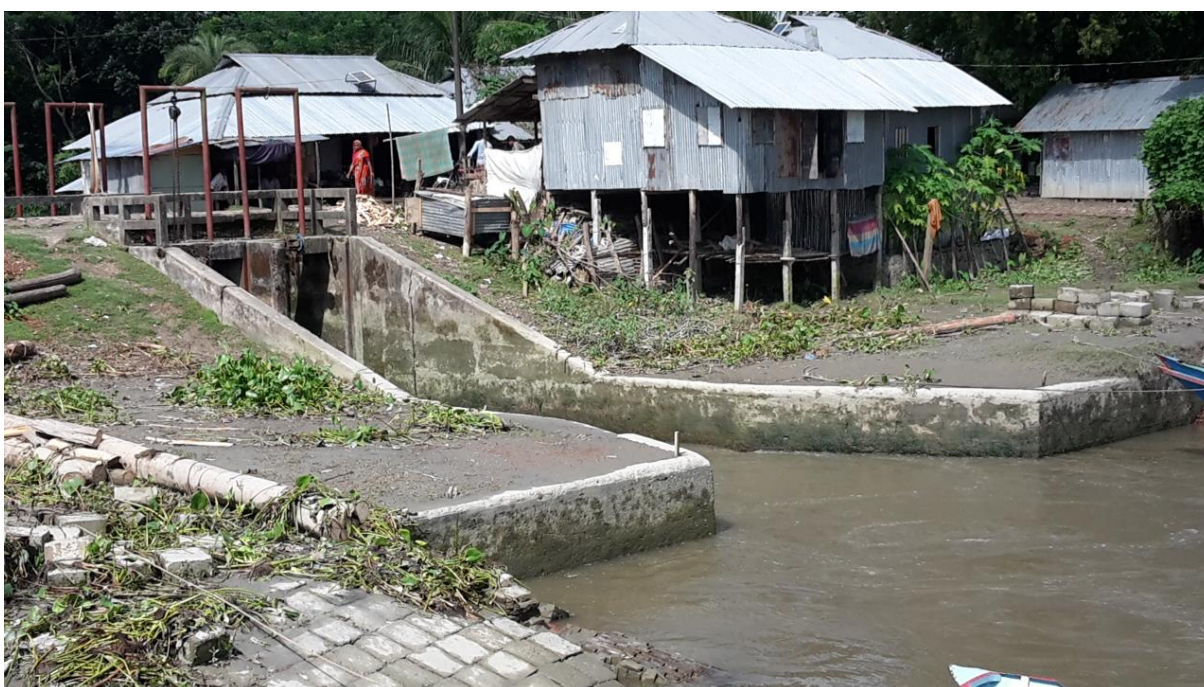
Picture 3.3: Amkhola drainage sluice (Golachipa river side)
