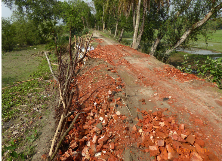
Figure 20: Low embankment section where carpeting has already started.
