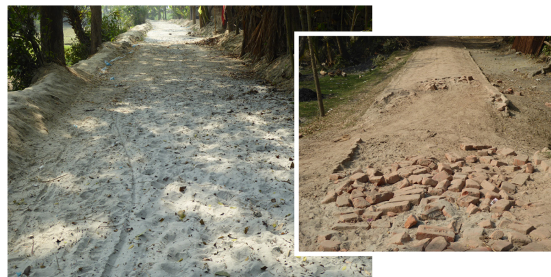
Figure 10: Earth and brick roads deteriorate rapidly and create many challenges to communication and transport
