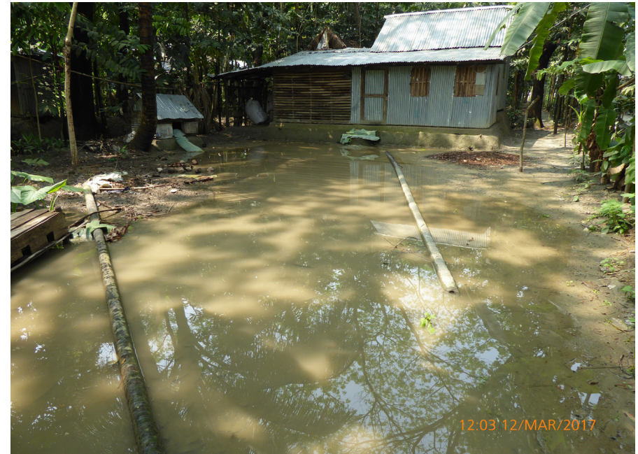
Figure 22: Drainage congestion around a house. This photo was taken in March 2017 during the dry season, 2-3 days after a rain event.
