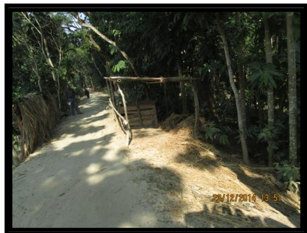
Figure 4: Tree Plantation on the slope of embankment at polder-43/2A
