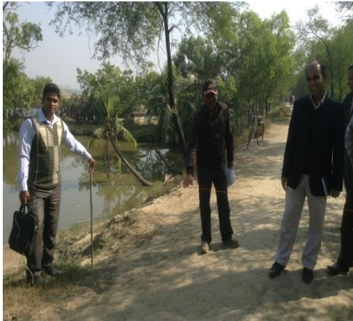
Deep Pond within Country Side Toe of Dike
