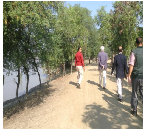
River within the Outside Toe of the Dike
