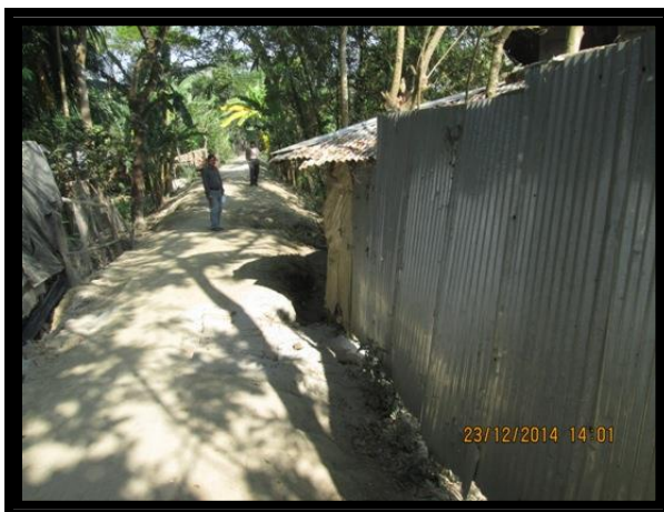
Figure 3: House constructed on the embankment at polder-43/2A
