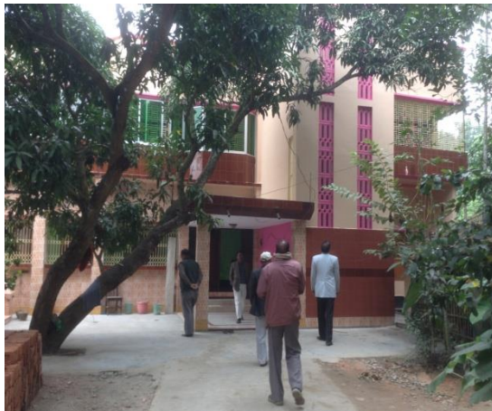
Front View of the Two Storied Building
