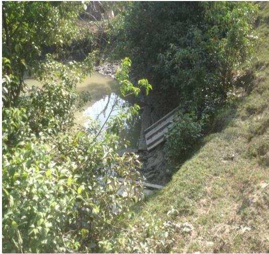
Private Outlet to be Replaced by Bigger Sluice
