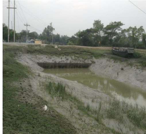
River Side Face of the Sluice, No Operation Deck
