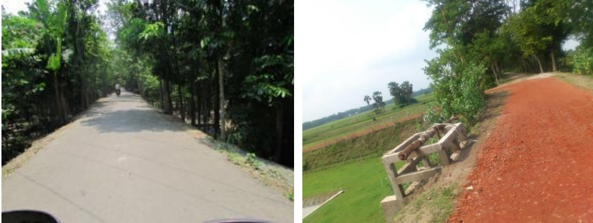
Photo 6.8: Soling and risk of damage to a paved road in the polder
