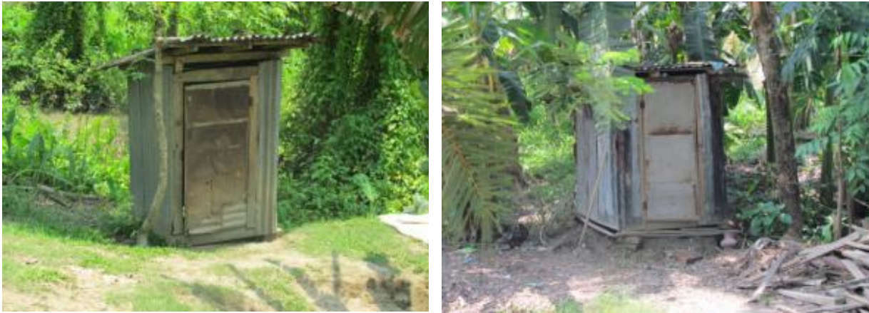
Photo 6.6: Sanitation facilities in the polder area
