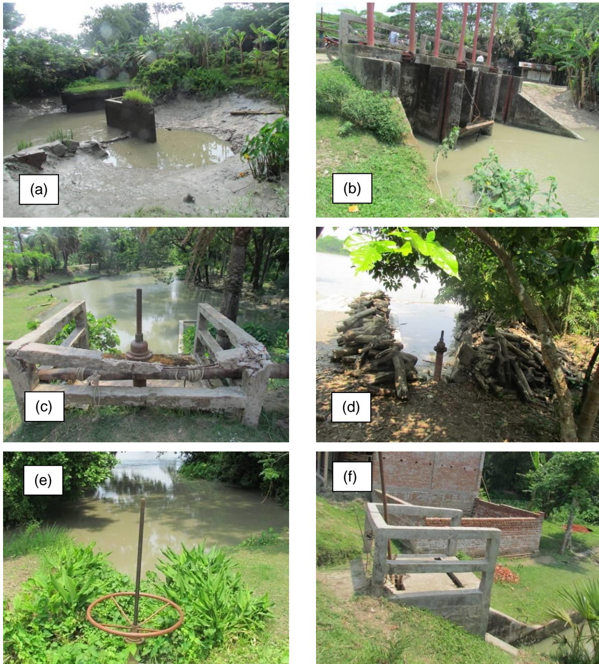
Photo 4.2: Existing status of sluiice gates
