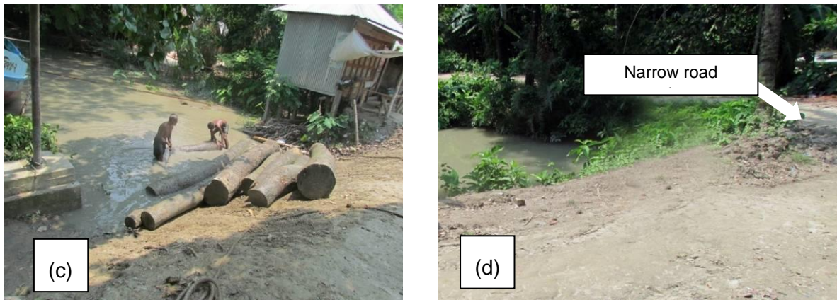
Photo 4.1 : Existing status of embankment
