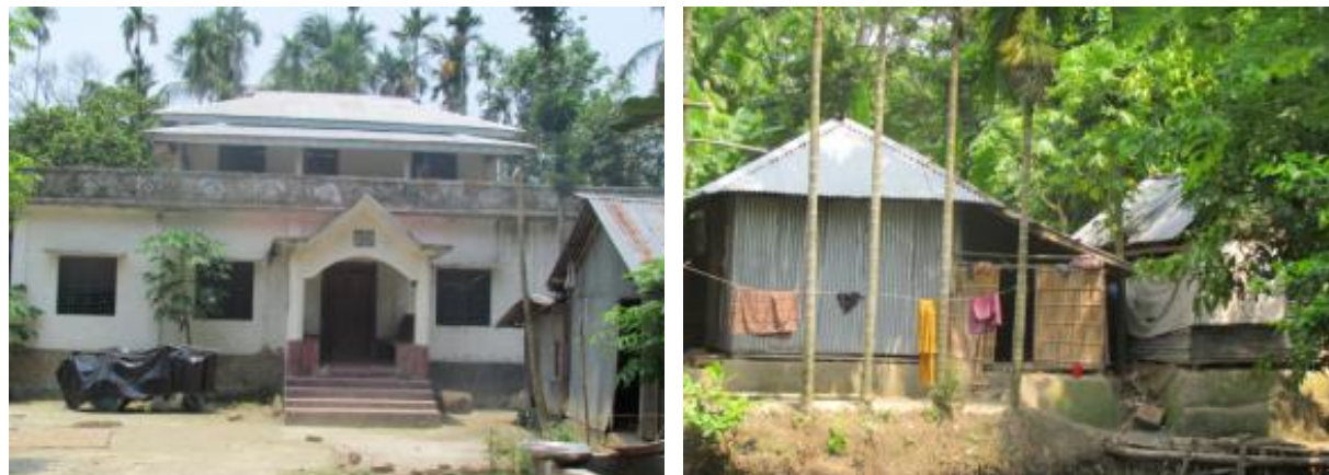
Photo 6.5: Housing structure in the polder area
