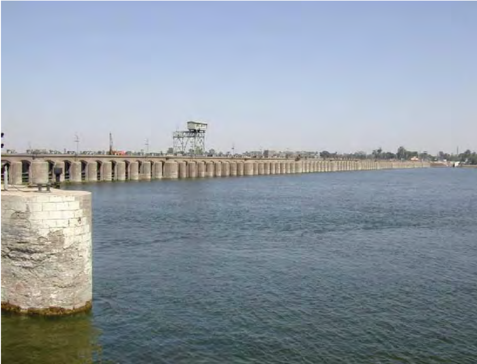
Assiut Barrage View from Upstream
