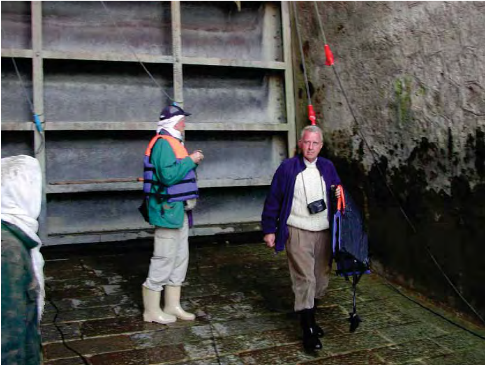
Assiut Barrage Vent Dewatering and Inspection
