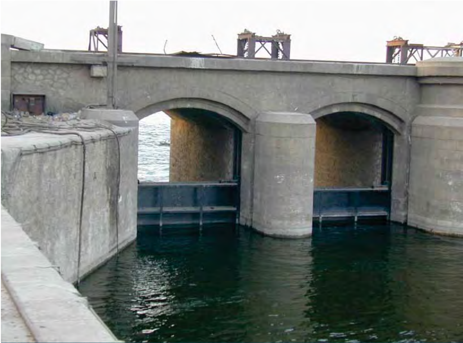
Assiut Barrage Gate Bays from Upstream
