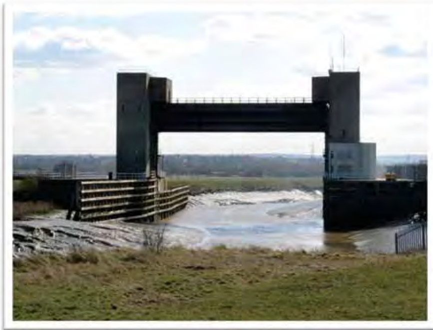
Dartford Creek Barrier
