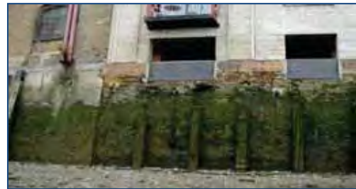
Masonry gravity walls
