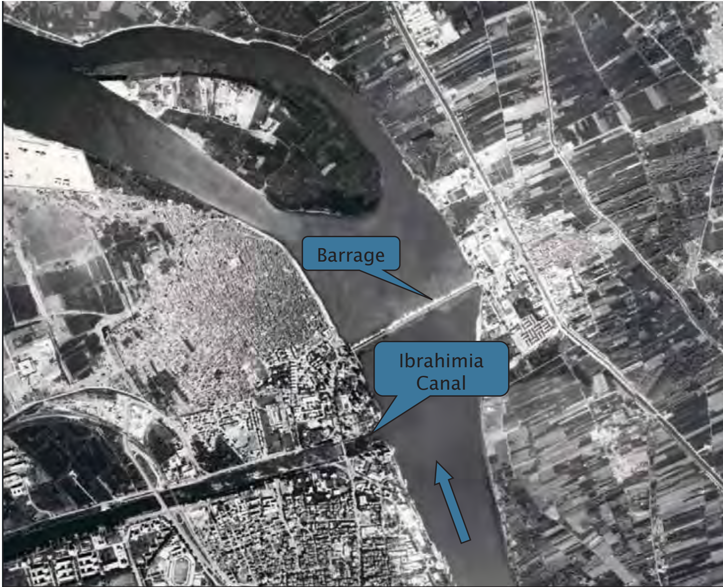
Assiut Barrage Aerial View
