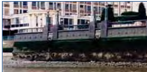
Concrete gravity walls
