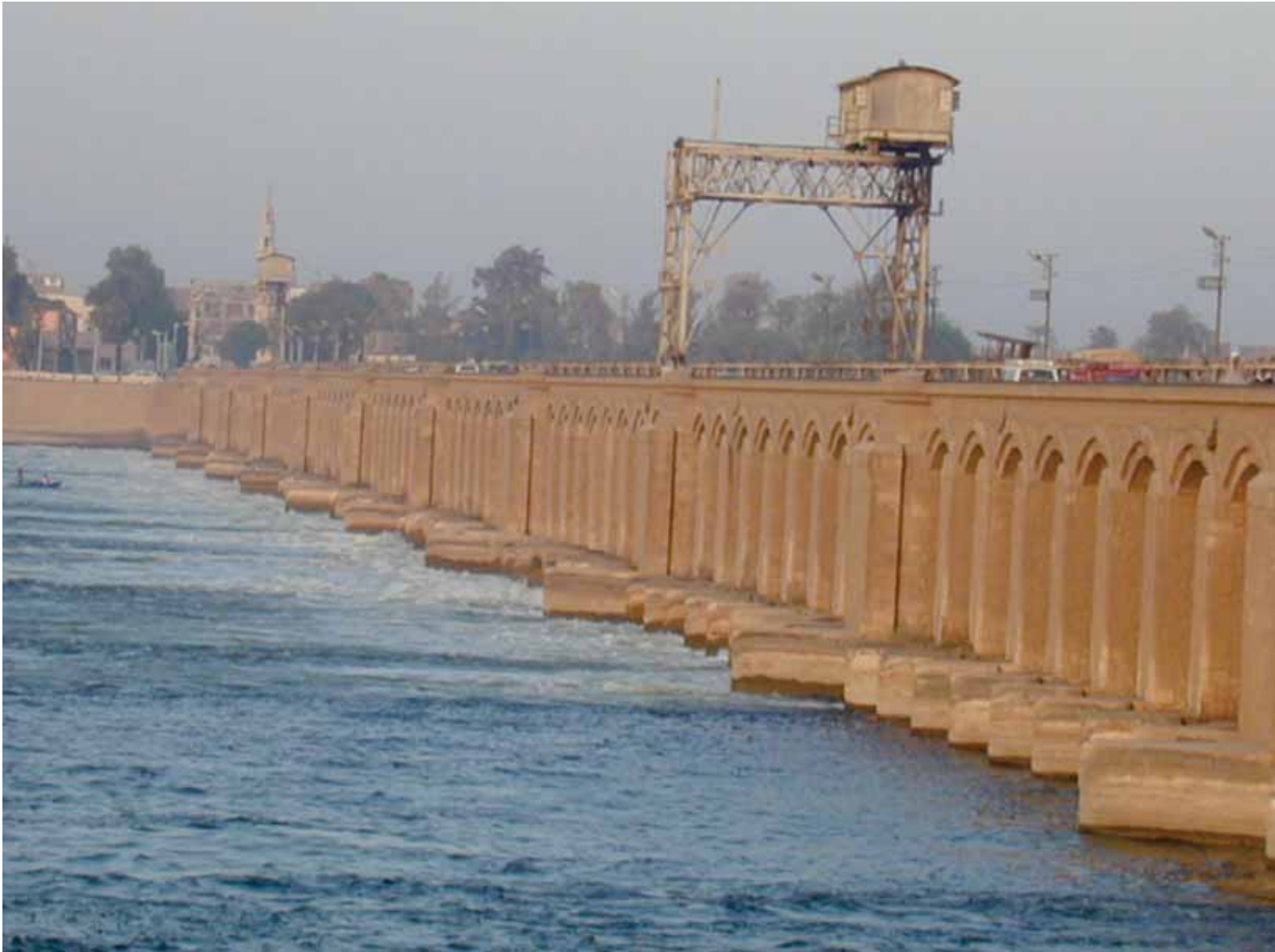
Assiut Barrage View from Downstream
