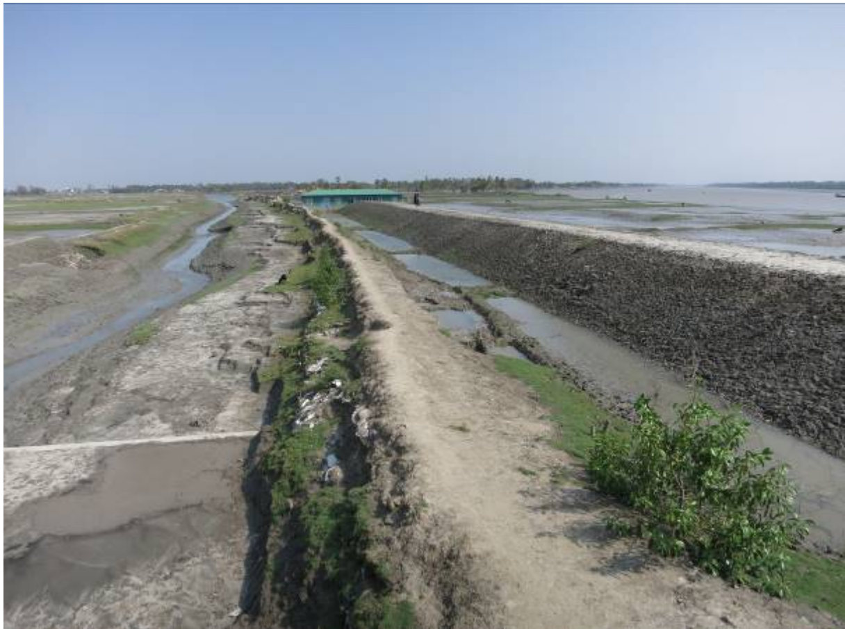
Figure 3-6 School building (in background) preventing the completion of the new embankment (to the right) with the emergency embankment in the center close to a major drainage khal on the left
