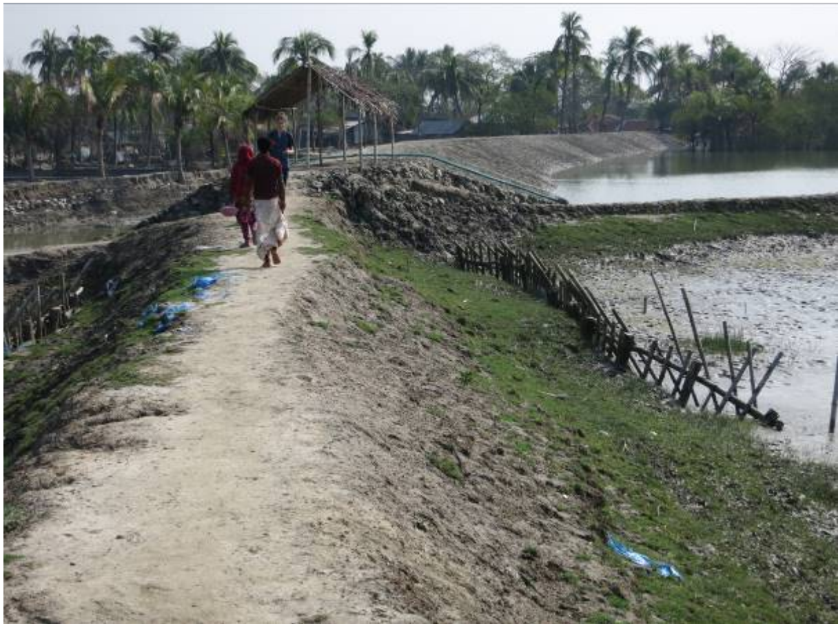
Figure 3-2 partial closure of upstream breach without attaining the final crest level
