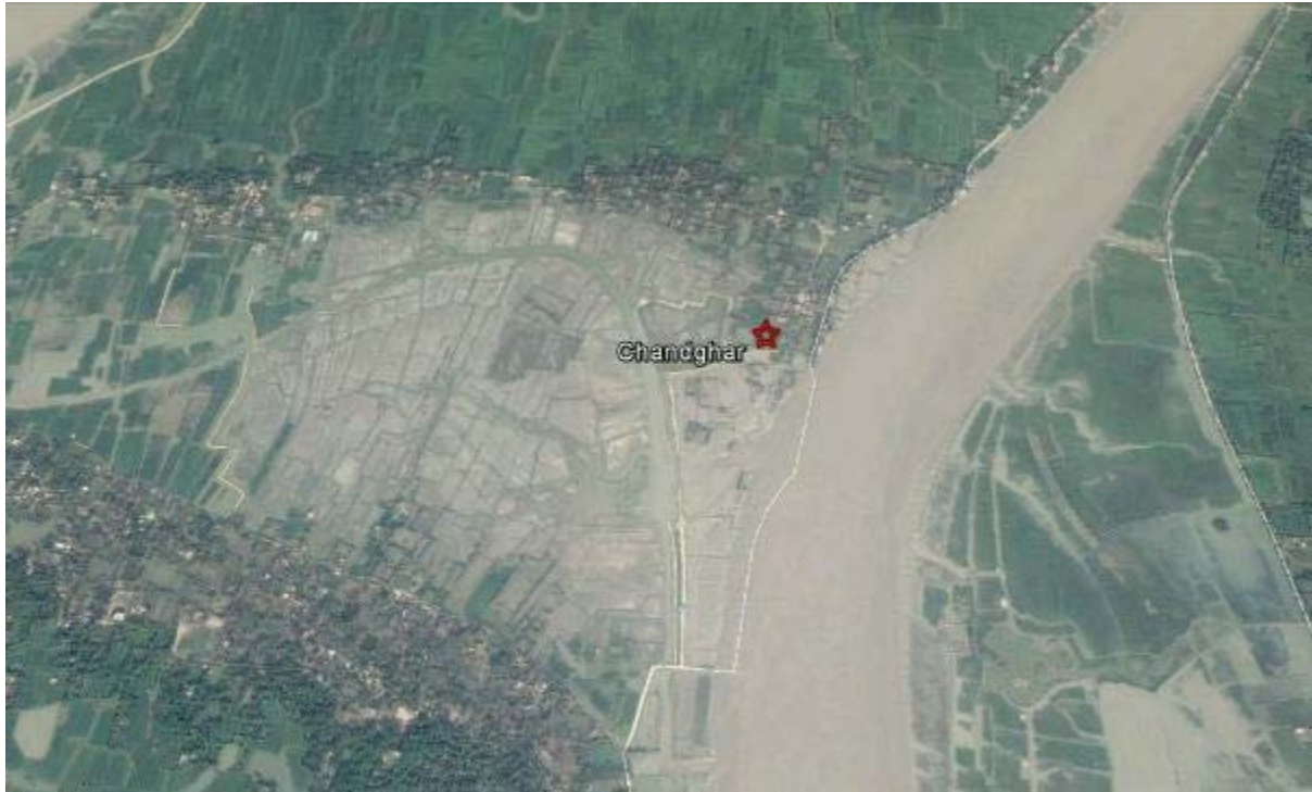
Figure 1-1: Areal view of the Chandghar area of Polder 29, where the embankments breached (Image from Google Earth, November 15 th , 2016)
