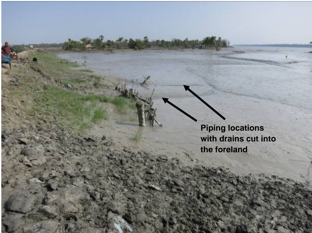
Figure 3-4 Piping through the embankment (riverside view)
