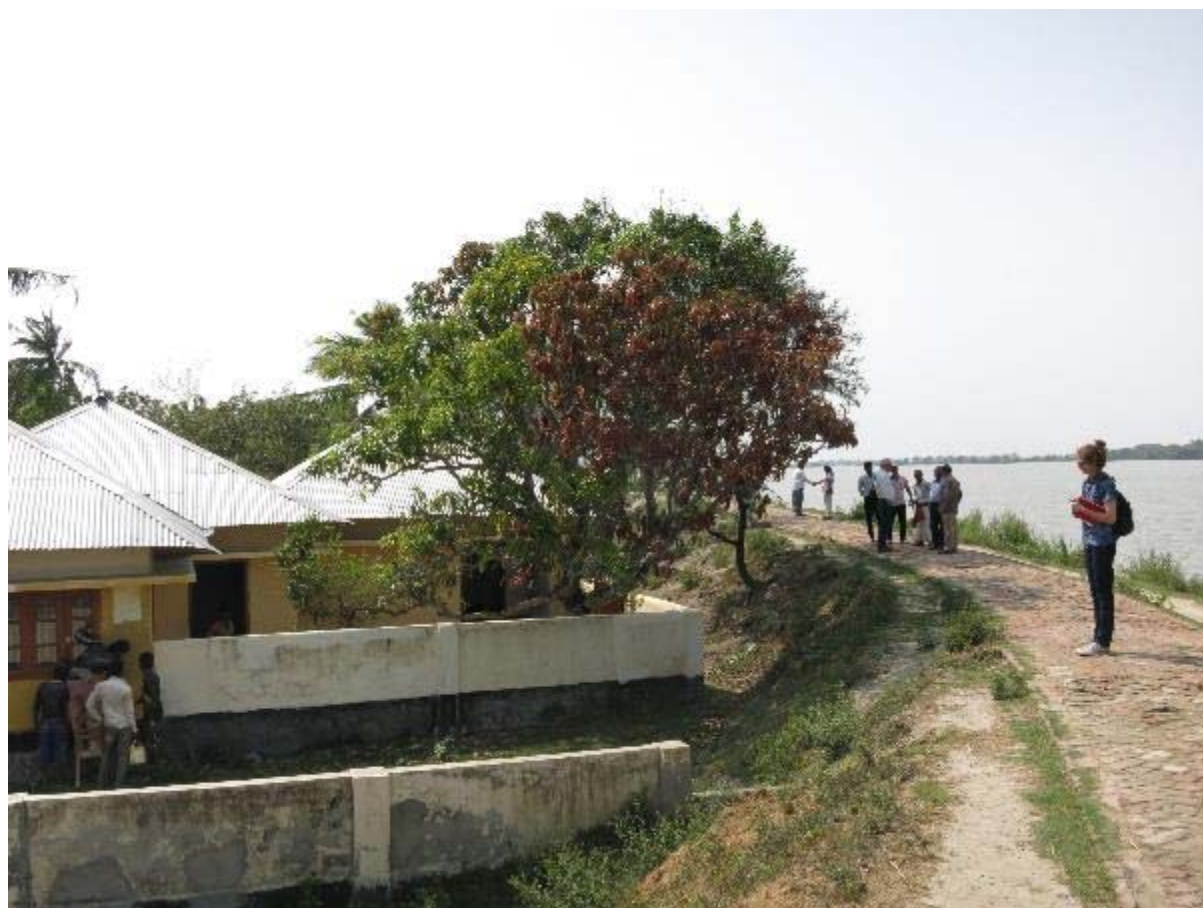
Figure 3-11 Training center of Polder 29 under rehabilitation with earlier realigned embankment
