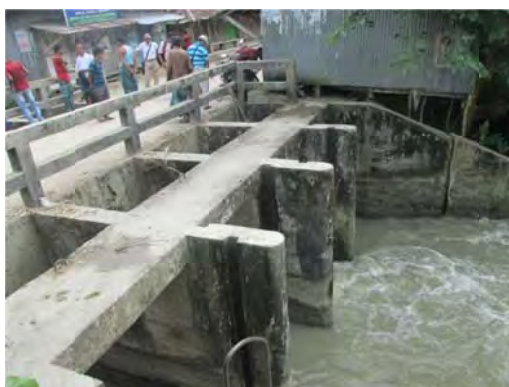
Picture 2.9: Chadpura Drainage Sluice of Polder 55/2C
