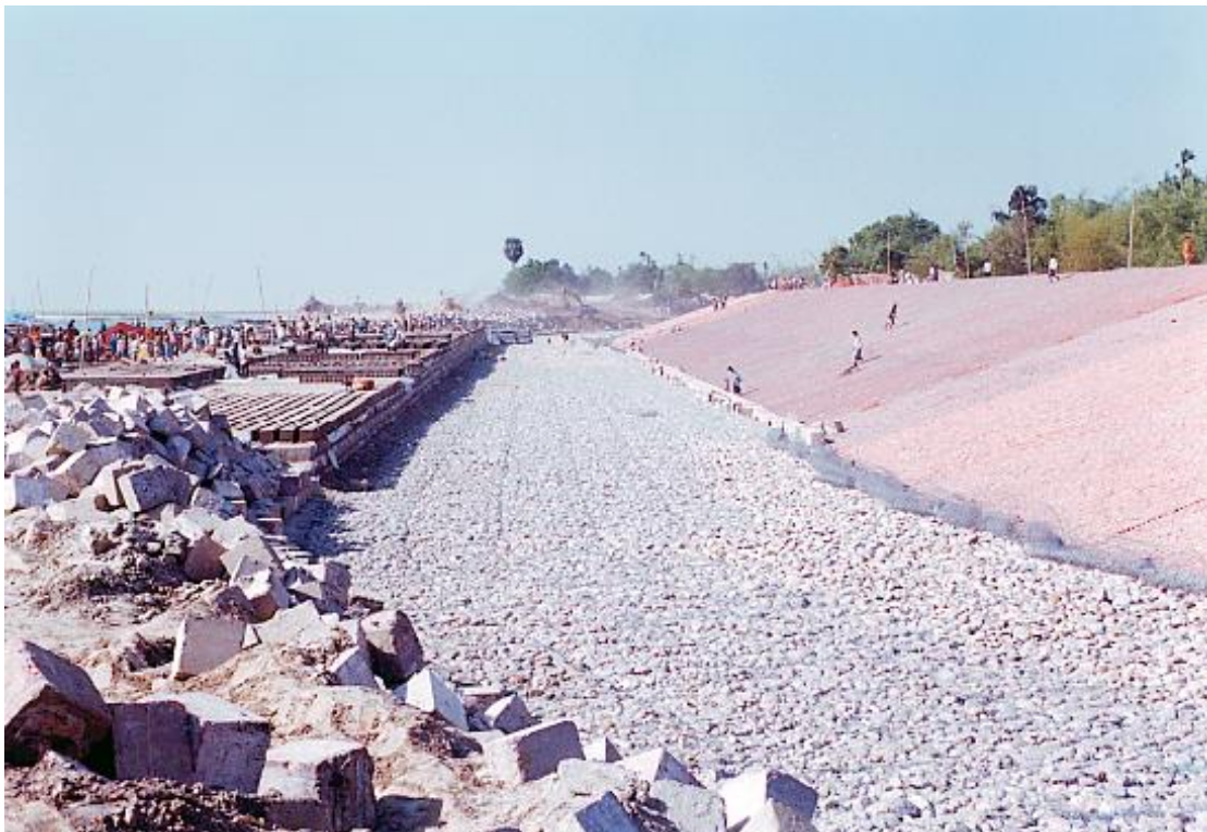
Figure A.6 Revetment along Jamuna River at Ghutail.
