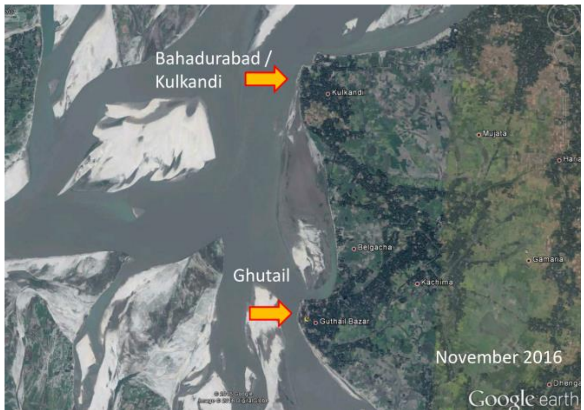
Figure A.8 Revetments at Bahadurabad / Kulkandi and Ghutail along Jamuna River intact after 20 years (source: Google Earth).
