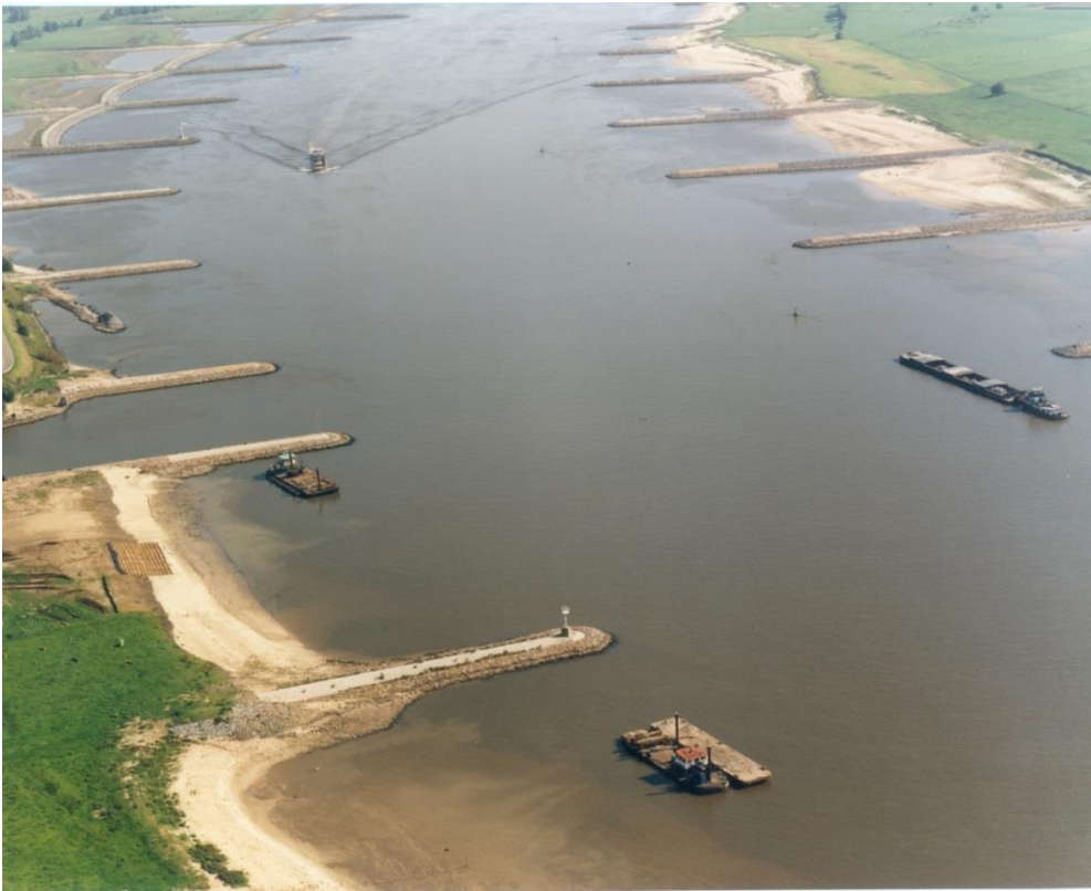
Figure A.2 Normalized river in the Netherlands with groynes to establish a uniform width.
