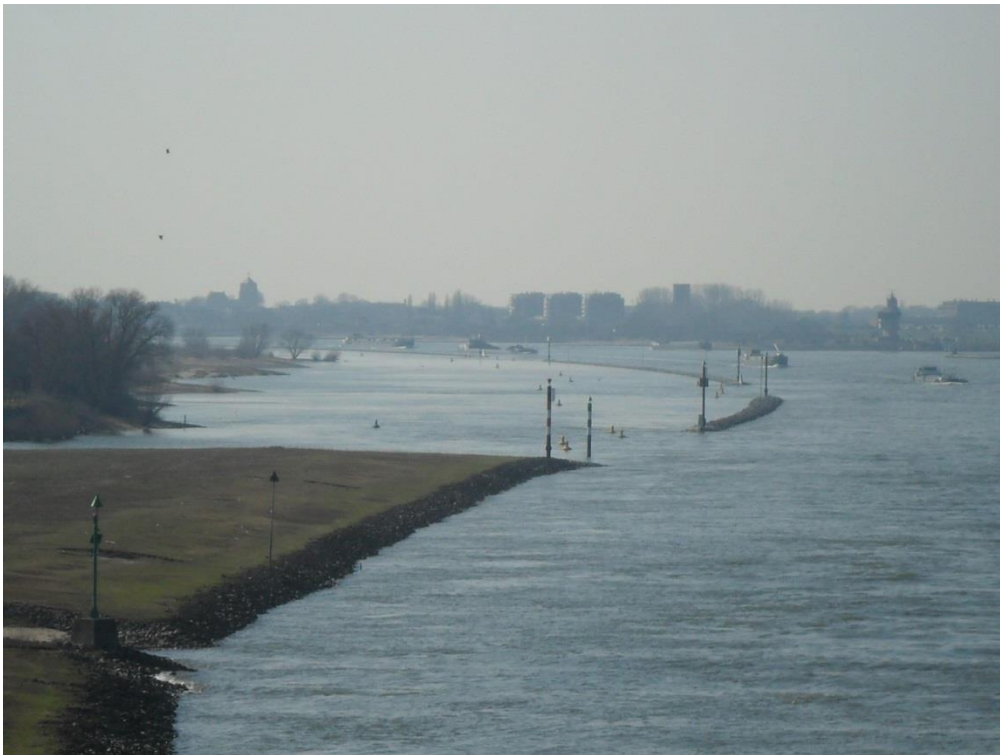
Figure A.3 Longitudinal training dams on the river Waal in the Netherlands.
