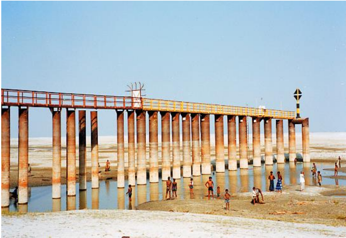
Figure A.5 Permeable groynes along Jamuna River at Kamarjani.
