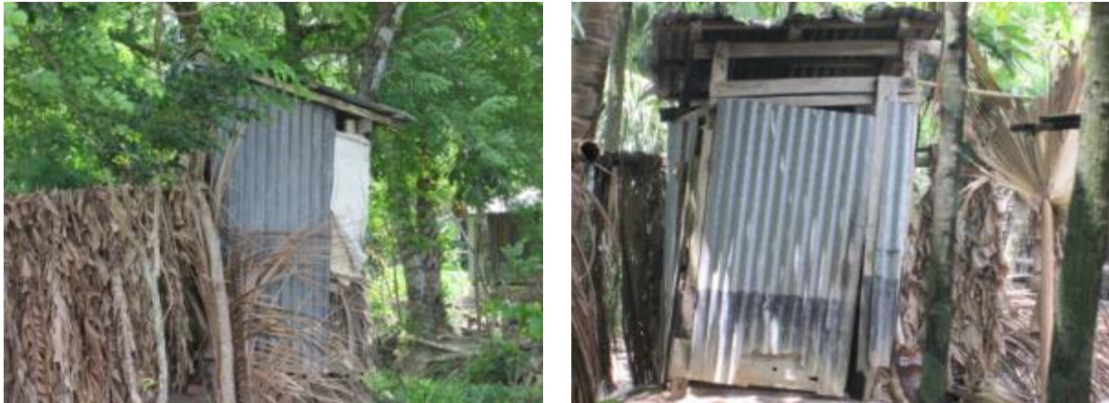
Photo 6.4: Sanitation facility in the polder area
