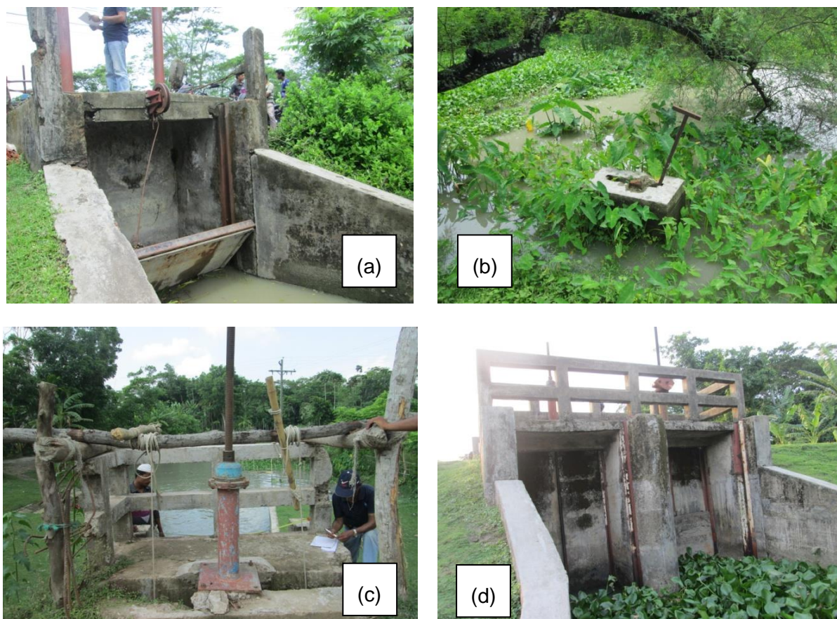
Photo 4.2: Existing Status of Sluice Gates
