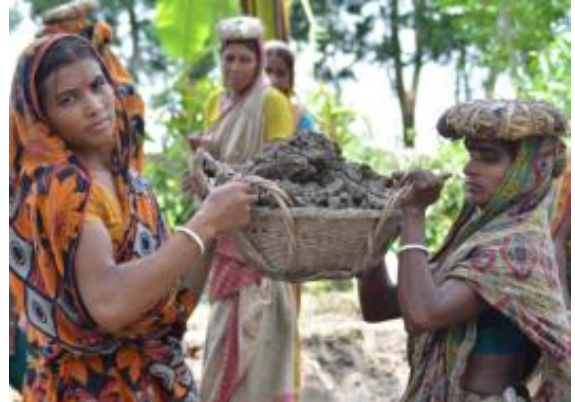
earthworks by LCS, Patuakhali, June 2014
