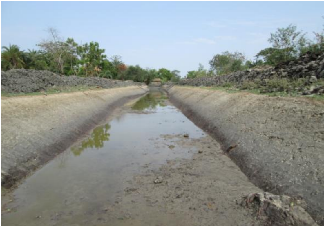
Figure 2: Canal Re-excavation in Polder 22
