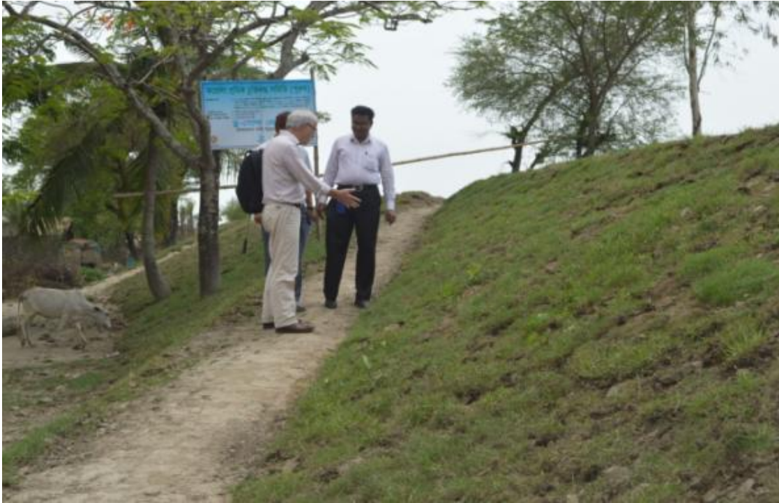
Figure 1: Embankment Re-sectioning in Polder 22
