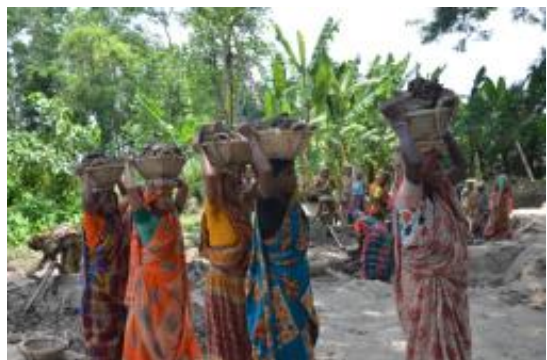
earthworks by LCS, Patuakhali, June 2014
