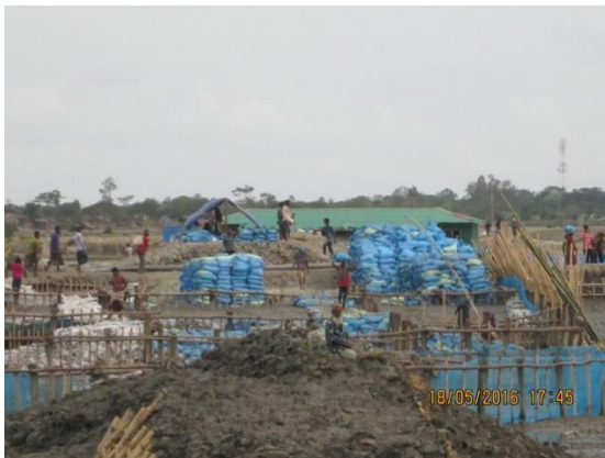
Figure-18: Sand Filled Synthetic Bags for Cross Dam -3
