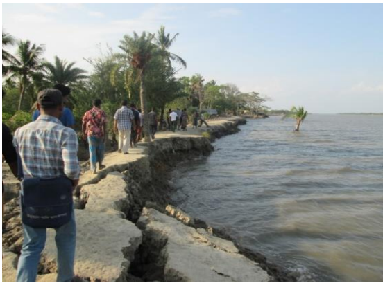
Figure-11: Severe Erosion – on the Verge of Failure
