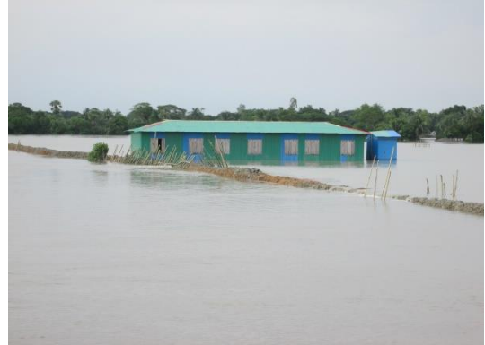
Figure-14: Flooded and Damaged Ring Dike
