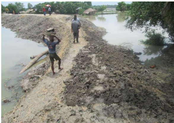
Figure-7: Under-Construction Embankment (not full section)
