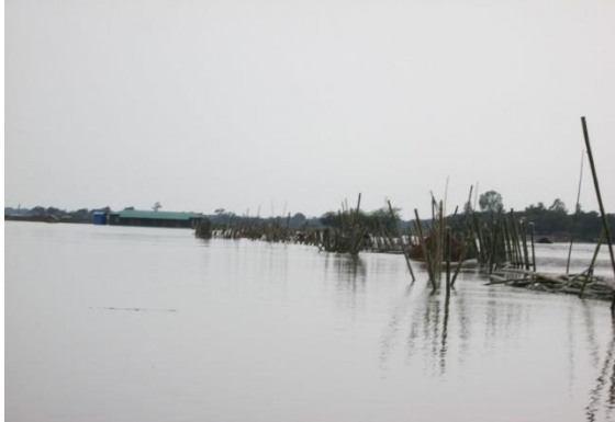
Figure-13: Rows of Bamboo Pins to Make Ring Dike
