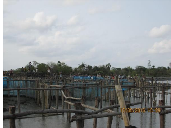
Figure-17: Wooden Bandaling for the Third Breach (Cross Dam-3)
