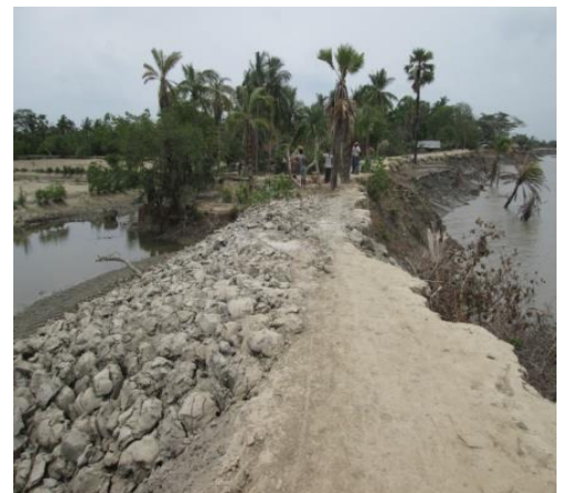
Figure-5: Backing of Embankment-Local Initiative
