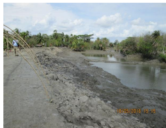
Figure-19: Under-construction Embankment
