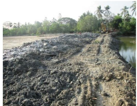
Figure-8: Under- Construction Embankment (Base Layer)
