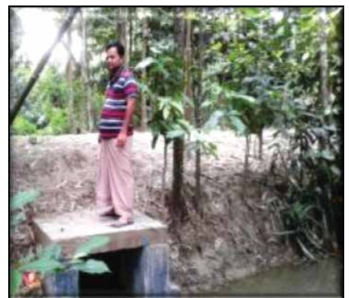
One of the Culverts constructed by UP
