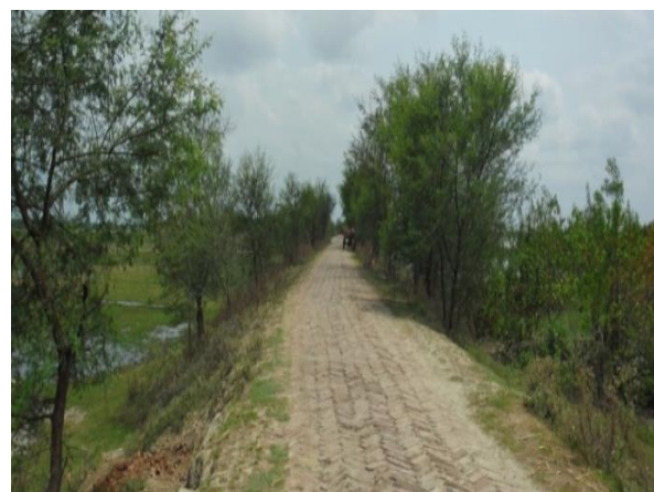
Photo 5.12: Rows of Babla and Sirish Tree along the Embankment Sides at the Polder
