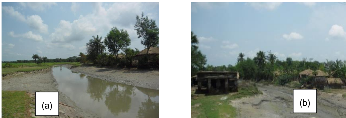
Photo 4.4: Narrow and Silted up Khals (a) Batiaghata khal, (b) Mailmara khal
