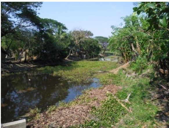
Photo 5.13: Internal Canal occupied by Free Floating Plant of Polder 30
