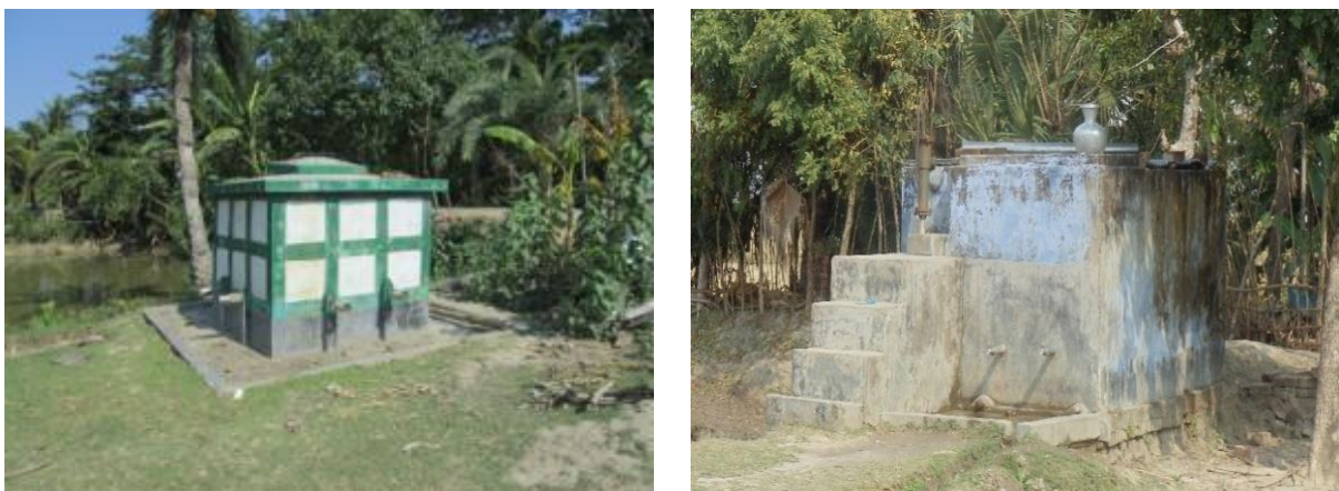
Photo 6.8: Community Level PSF
