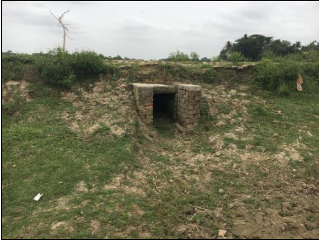
Figure 6: First culvert connecting WMU 1 and WMU 2
