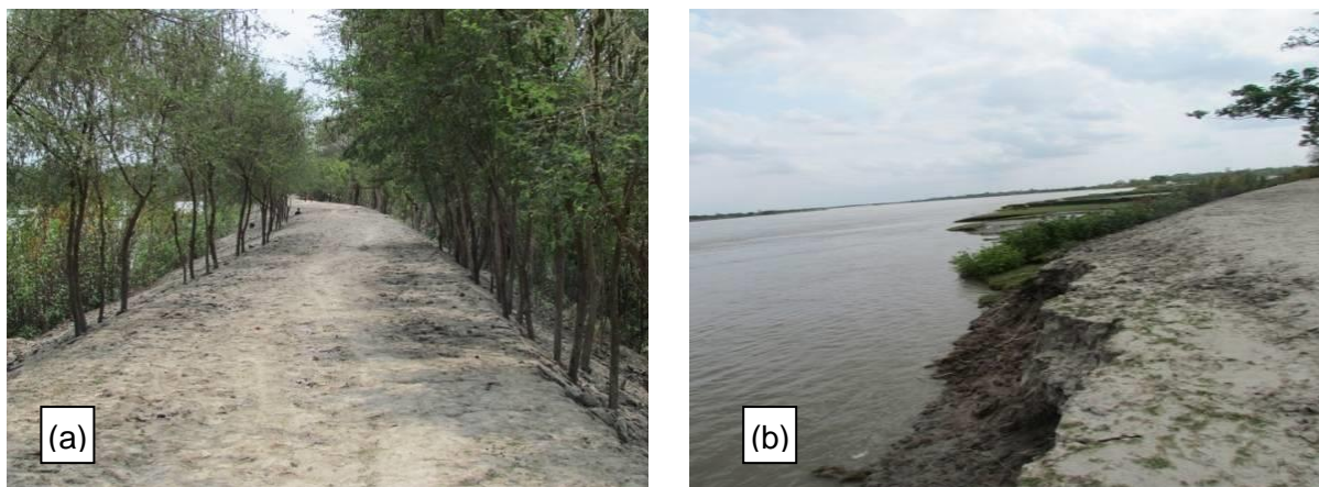
Picture 4.1: Existing Status of Embankments
