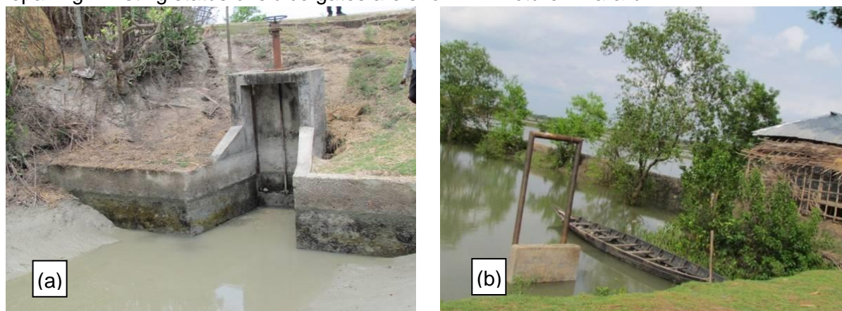
Picture 4.2: Existing Status of Sluice Gates
