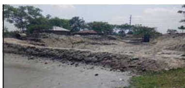
Cross Dam at Shalley Sluice Point
