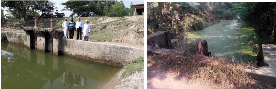
Photo 4.2: Existing Status of Sluice at Polder 55/2C
