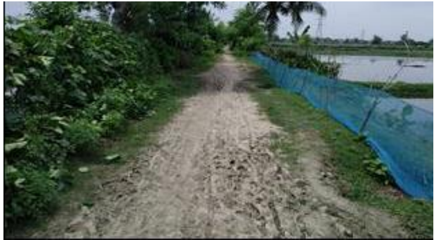
Photo 4.1: Existing Status of Embankments
