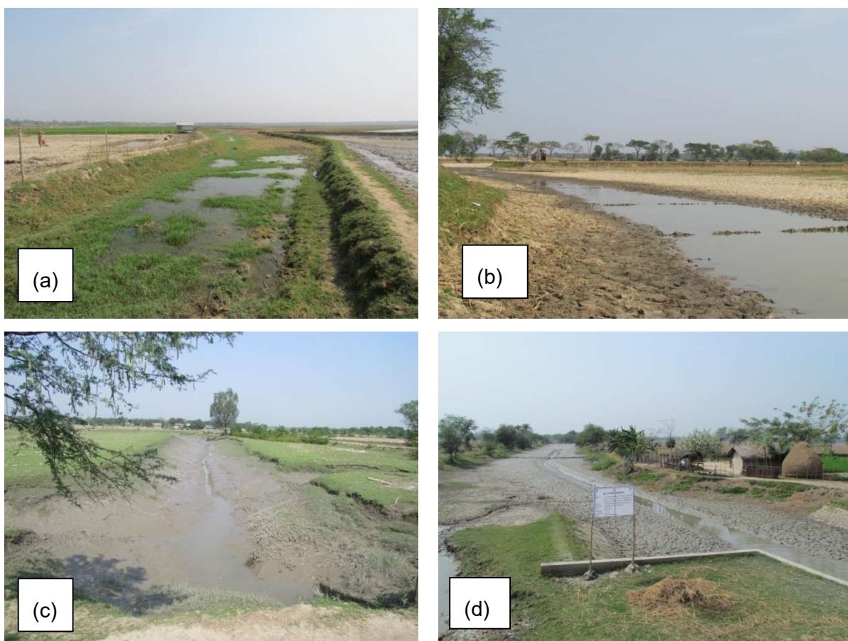
[(a)Silted up course along the Aro khal, (b)Narrow course of Asannagar khal, (c) Very narrow course of water at Golaimari khal, (d) Silted up bed of Kata khal]
