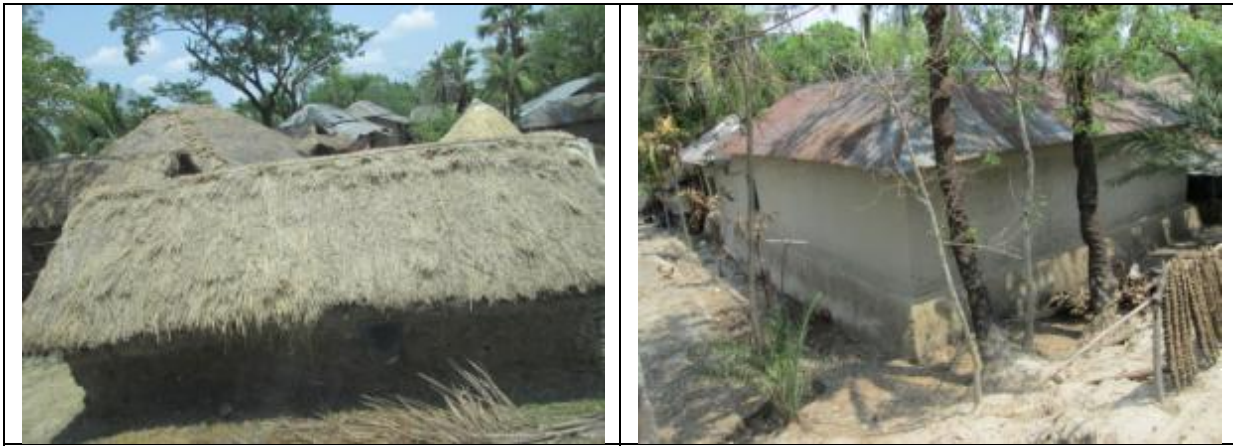
Photo 6.3: Jhupri House Photo 6.4: Kutch House
