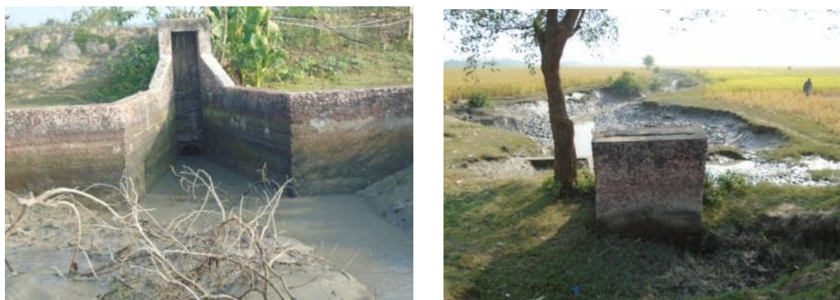
Photo 4.2: Existing Status of Narayankhali Sluice and Shialidanga Sluice at Polder 34/2
