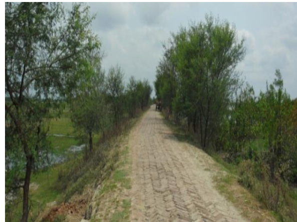
Photo 5.12: Rows of Babla and Sirish Tree along the Embankment Sides at the Polder
