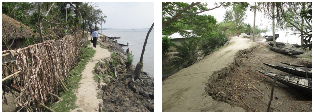
Photo 4.1: Existing Status of Embankments
