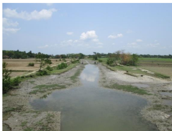
b. Baroikatakhal khal (Silted Up)
