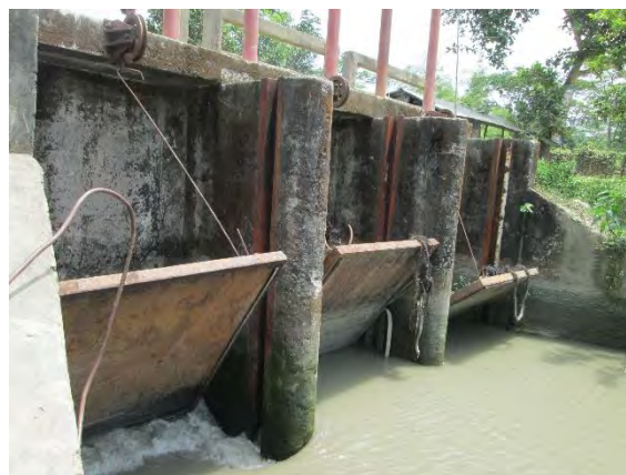
Figure: Flap gate of Gojkhali Sluice
