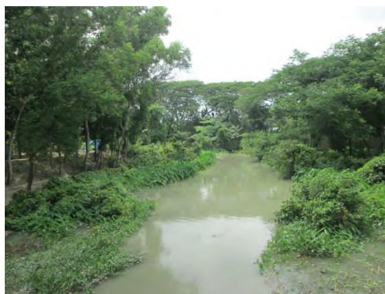
Figure: Outfall of Gulbunia catchment
