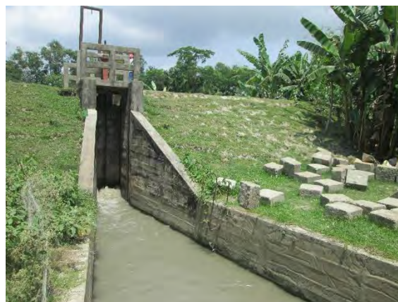
Figure: R/S of Doachara Sluice
