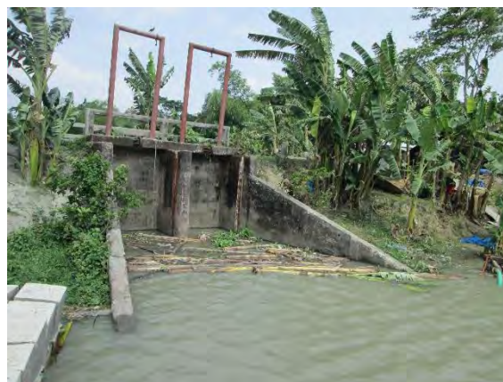
Figure: R/S of Dalachhara Sluice
