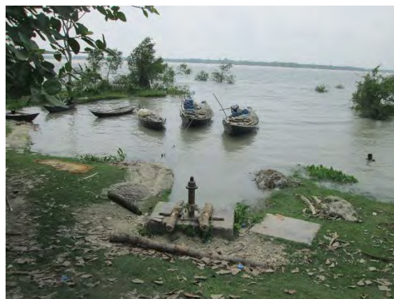
Figure: R/S of Kanta Sluice
