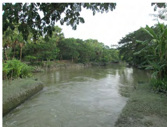
Figure: Outfall of Amtola catchment
