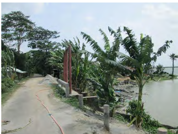
Figure: On-going Block pitching work of Dalachhara Sluice
