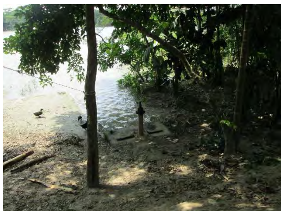
Figure: R/S of Debpur Sluice
