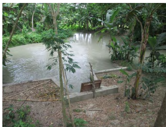
Figure: Outfall of Kewabunia catchment
