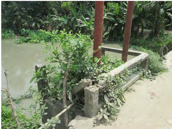
Figure: Khekuani Sluice
