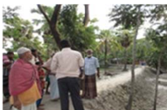
Dyke constructed by Balaikati WMG
