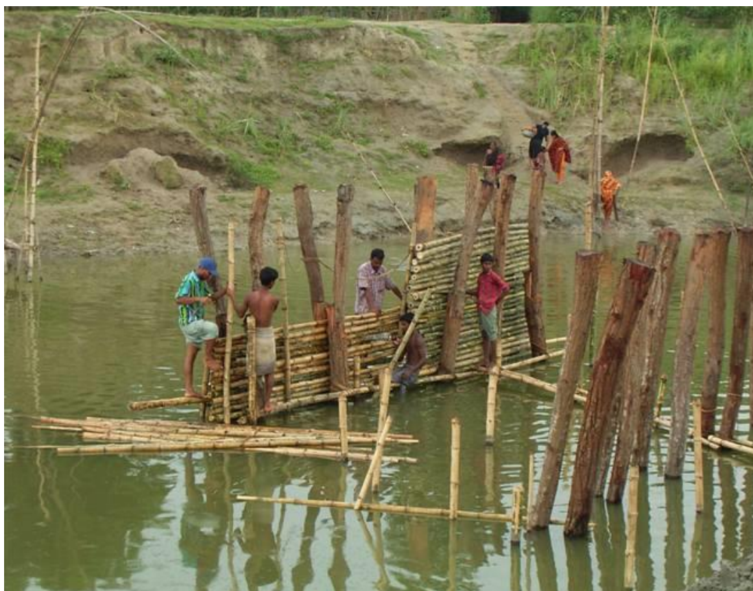
Figure 2.3. Bottom vanes under construction in the Elanjani river (Tangail).
