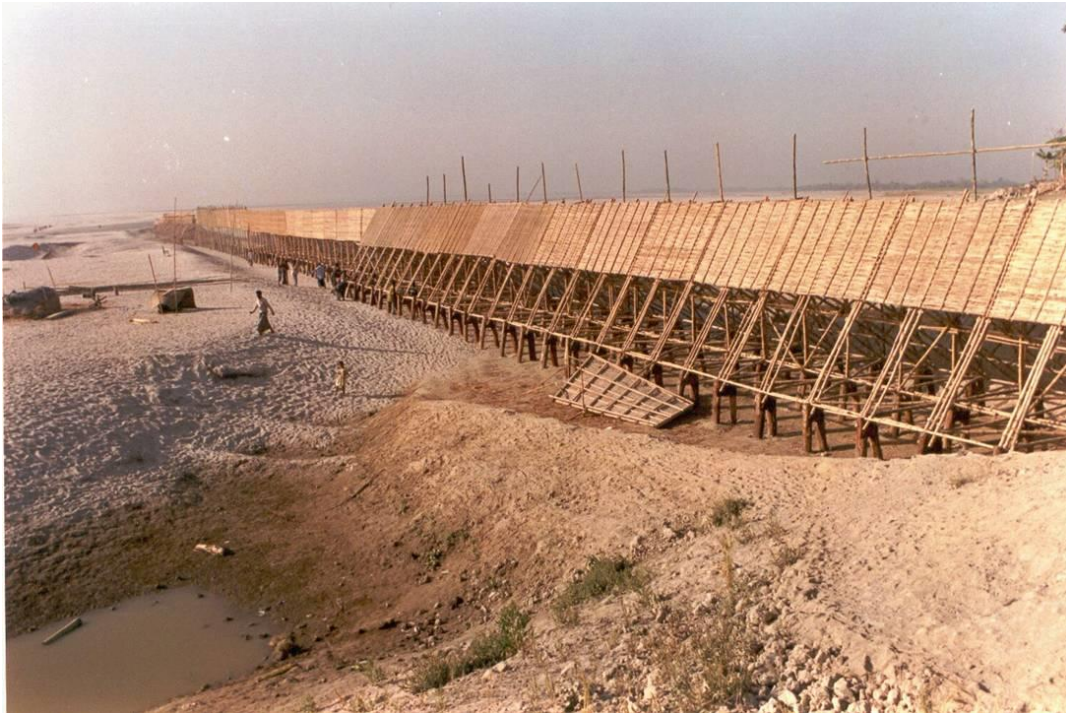
Figure 2.4. High-water bandal test structure in the Brahmaputra-Jamuna river at Katlamari.
