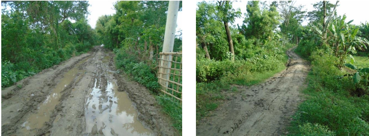
Photo 4.1 Existing Status of Embankments
