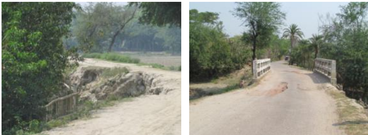
Photo 6.5 Road networks within the polder
