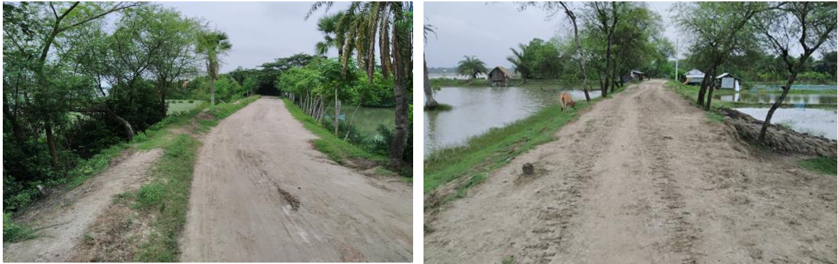
Photo 4.1 Existing Status of Embankments
