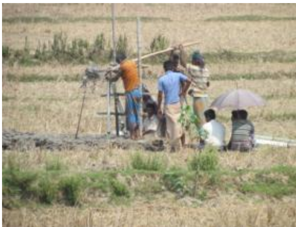
Photo 6.3 Installation of deep tube well at Vabagatipur
