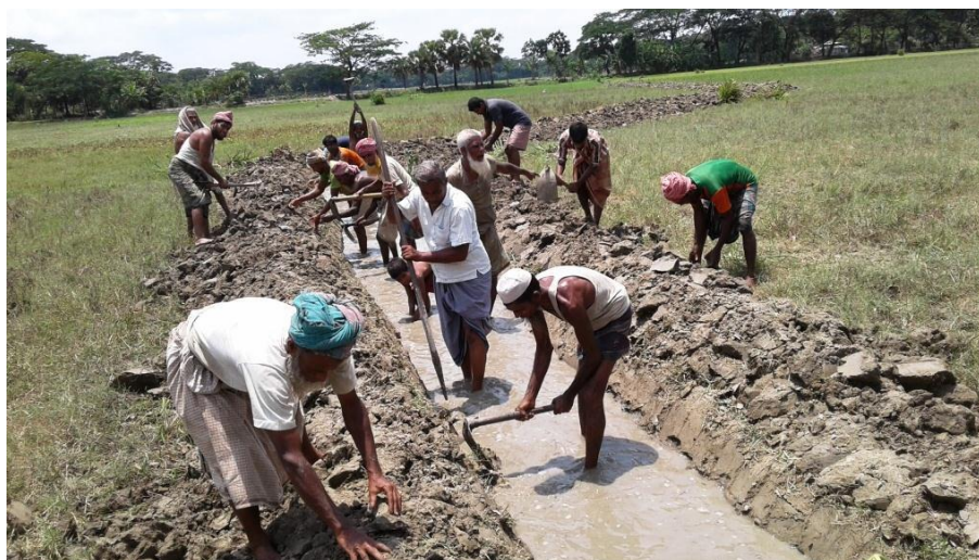
Figure 1: Dakshin Darandi WMG (P-55/2A) members are excavating drain
