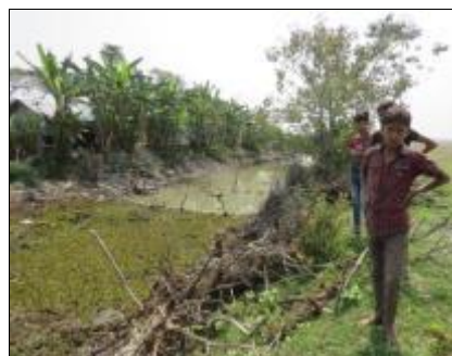
A dam over the mouth of the canal allows it to store sweet water
