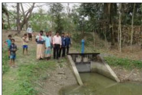
The community paid for half of this complex sluice gate
