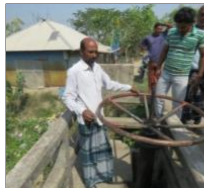
Powerful people no longer open the sluice gate at their whim. The sluice catchment area has gate operators
