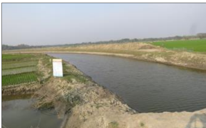
The re-excavated Amodkhali Canal allows a profitable rice crop to be grown
