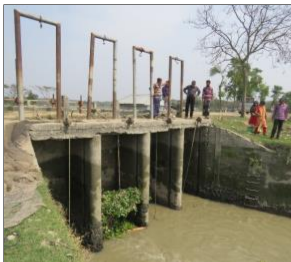
Taking ownership of the sluice gate
