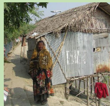
Figure: Deserted RE Electrification System
