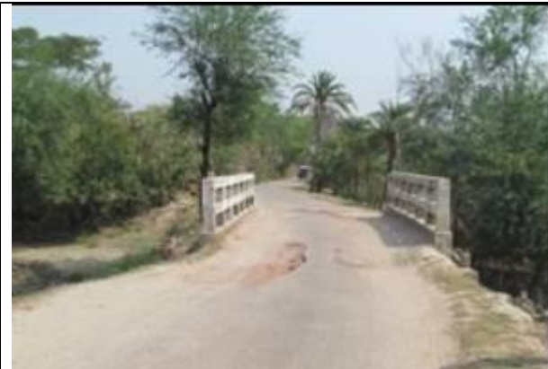
Photo 6.1: Road networks within the polder
