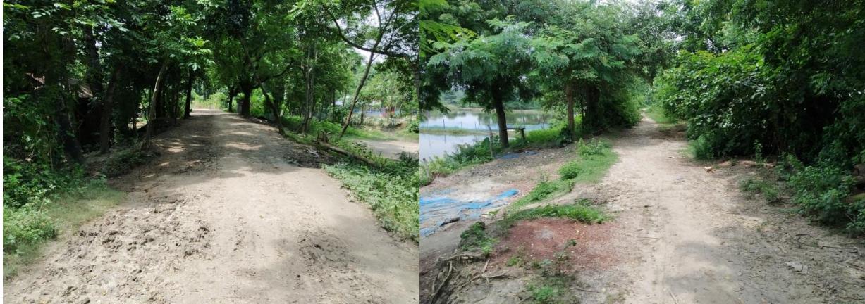
Photo 4.1: Existing Status of Embankments of polder 27 Water Control Structures
