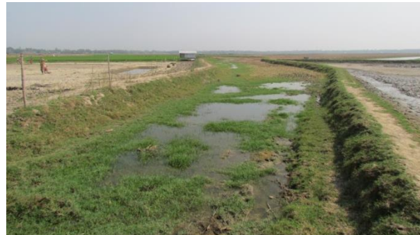
b. Kalatola Khal (Silted Up)
