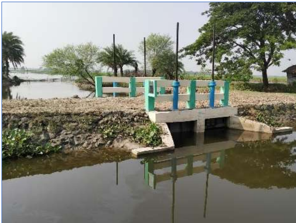
Picture 2: 2 vent gated culvert constructed at Gajendrapur CAWM area in polder 29, Khulna. 500 ha land will get benefits from this gated culvert.
