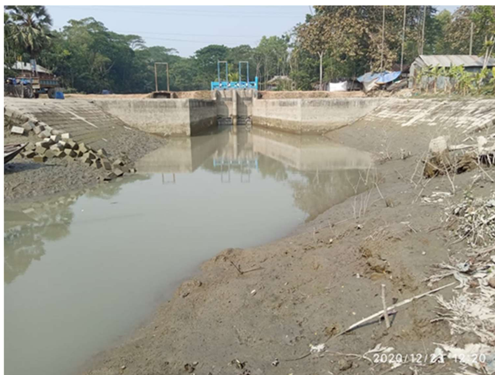
Picture 10: Re-construction of the Khekuani 2-vent regulator has been completed in polder 43/2F, Patuakhali. After the completion of this work, the water management and cropping intensity of this area has improved.
