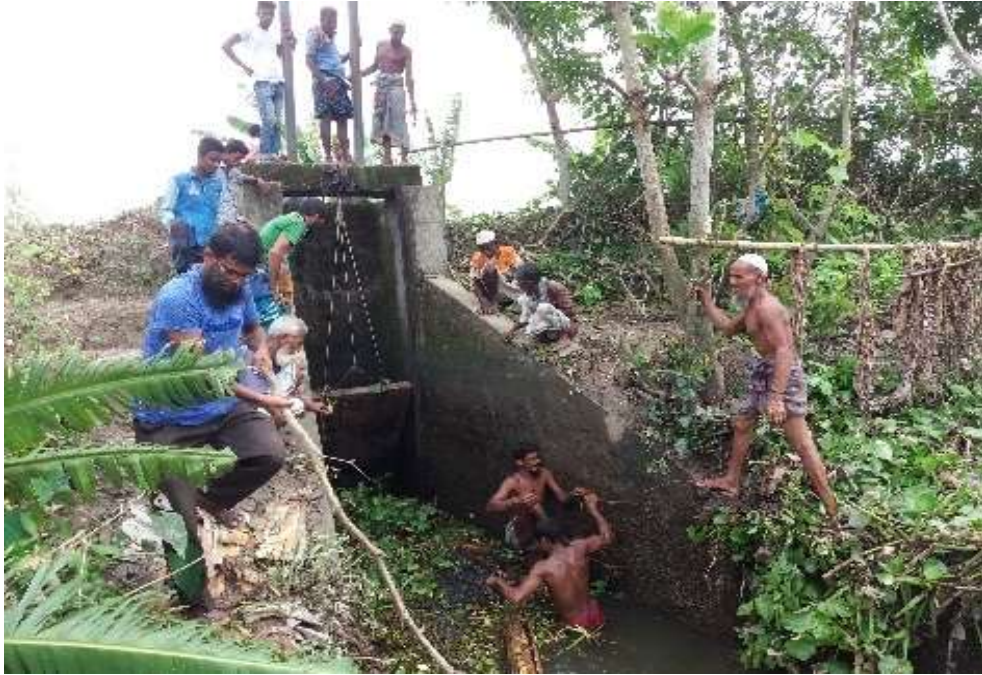
Picture 5: Two WMGs in polder 43/2D jointly removed silt from both sides of the sluice, cleaned the water hyacinth, and painted the sluice. The cost BDT 15,000 was shared by the two WMGs. As a result, the sluice operation becomes easily and lifespan has increased.
