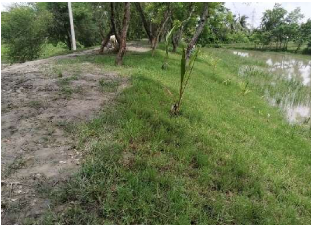
Picture 9: The embankment of the southern part of the polder-25, Khulna was low. After the embankment resectioning works, the area is now protected from the flood.
