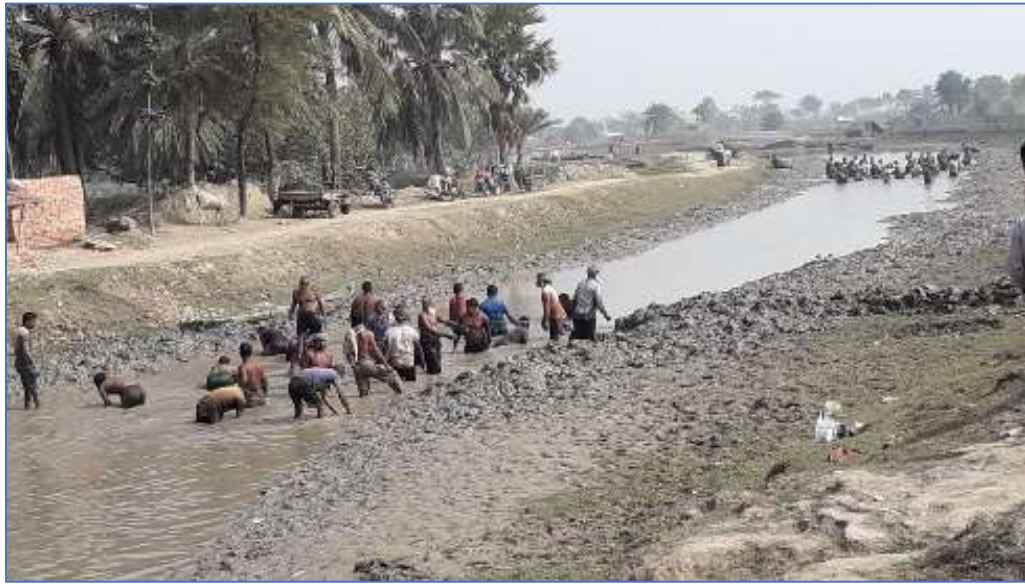
Picture 1: Chohera Catchment O&M Sub-Committee in polder 25 removed silt several times from sluice khal involving 403 self-contributory laborers to cultivate 800 ha of land under Aman and rabi crops which was supported by WMA, UP, and Upazila Parishad
