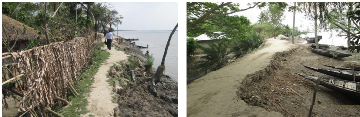
Photo 4.1: Existing Status of Embankments
