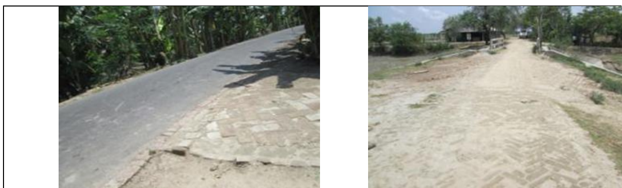
Photo 6.11: Paved and Soling Roads in the Polder Area
