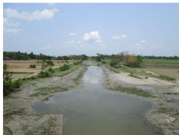
b. Baroikatakhali khal (Silted Up)
