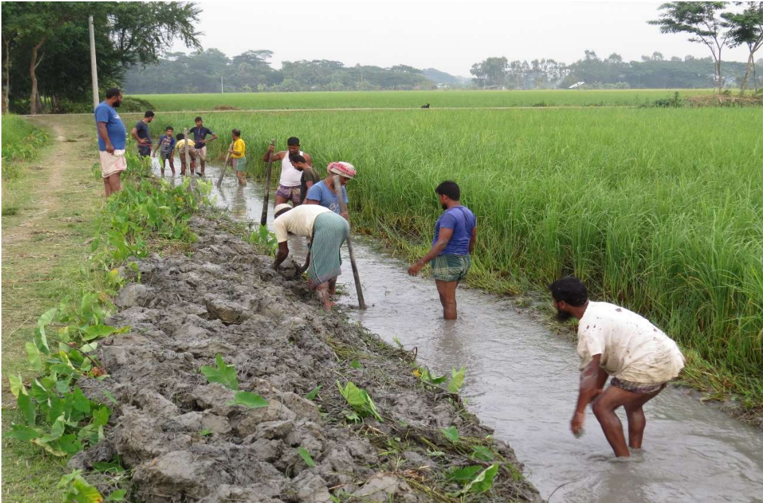
Photo 5: Excavation of drainage channel at 55/2A polder
