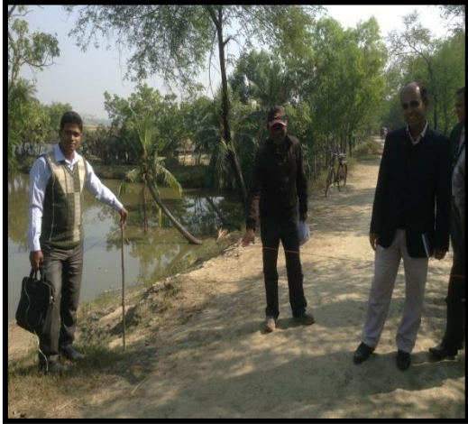
Deep Pond within Country Side Toe of Dike Side
