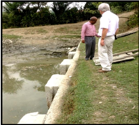
Wooden Fall Board on the Country Side of Sluice
