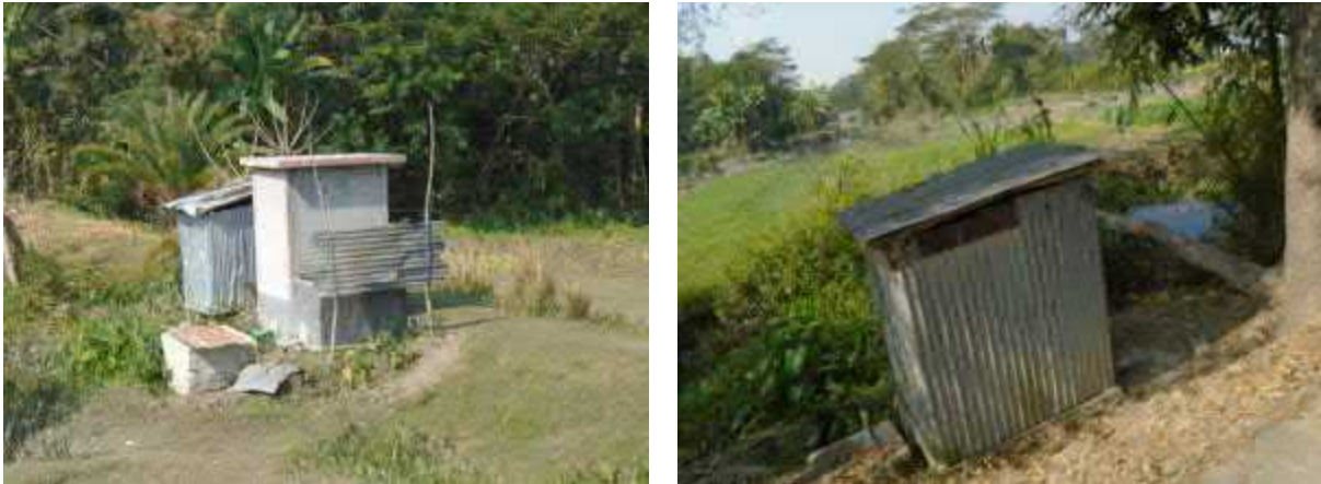
Photo 6.3: Sanitation facility in the polder area.
