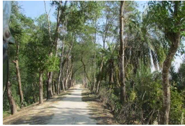
Photo 5.16: View of embankment side vegetation
