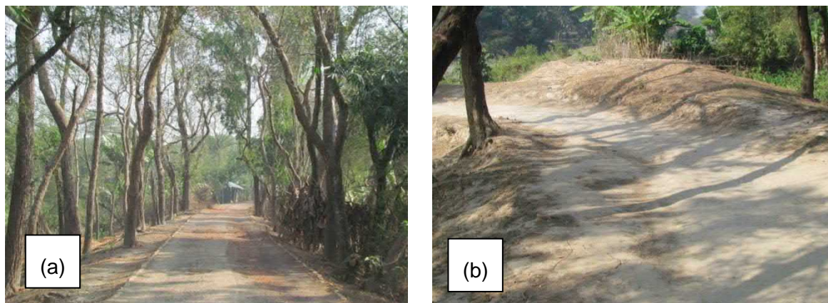
[(a)paved road surface at Sehakathi, suitable for various modes of transportation in all season, (b)unpaved road surface at Purba Jainkathi, which becomes slippery and unsuitable for communication in wet season]
