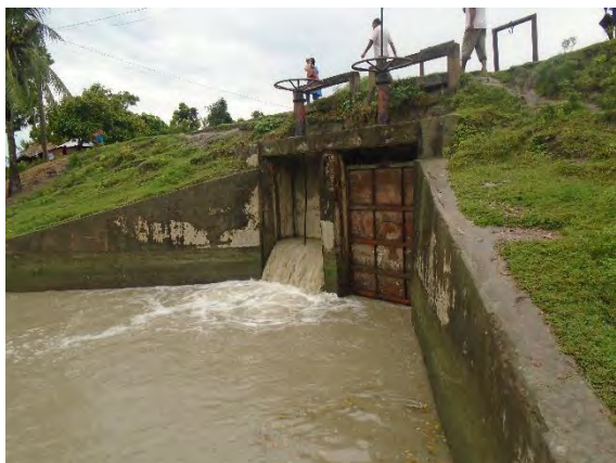
Figure: C/S of Chatchatia Sluice
