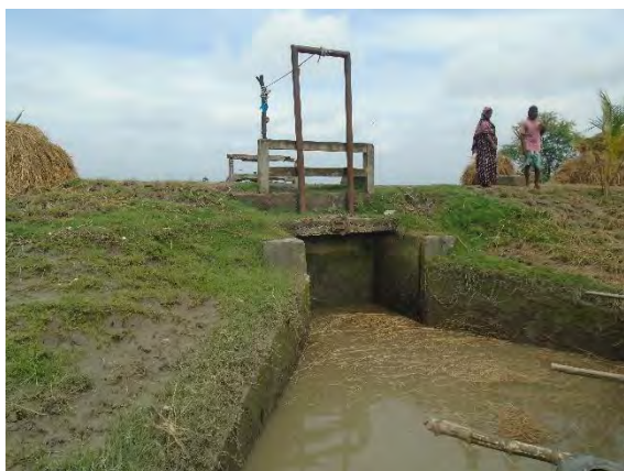
Figure: R/S of Ratankhali Sluice
