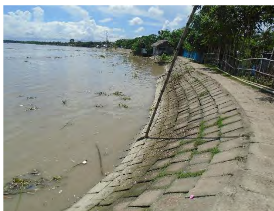
Figure: Bank protective work at Botiaghata
