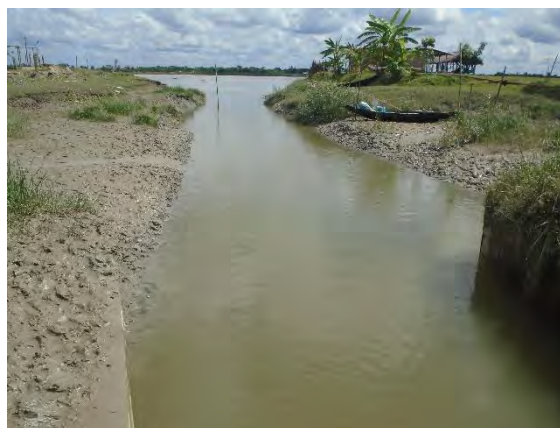
Figure: Outfall of Kismat Fultala Sluice
