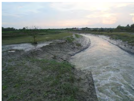
Figure: Outfall of Parbotiaghata catchment
