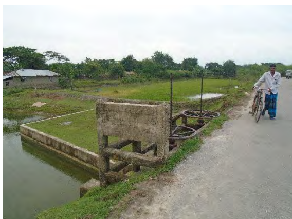
Figure: Telikhali (Old) sluice
