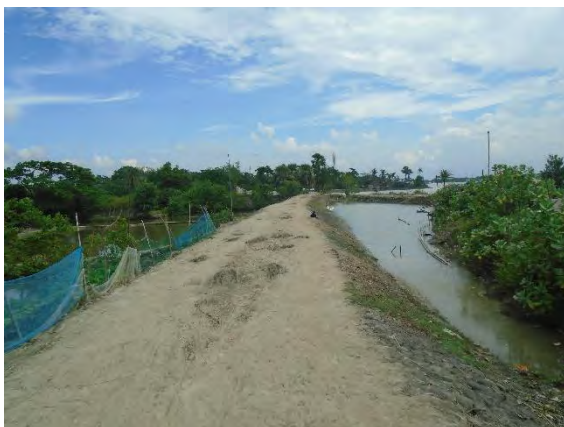
Figure: Retired embankment at Baro Auria
