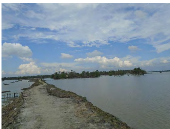
Figure: Retired embankment at Chadghar/Jalilakhali
