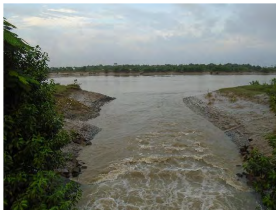
Figure: Outfall of Kanchannagar catchment
