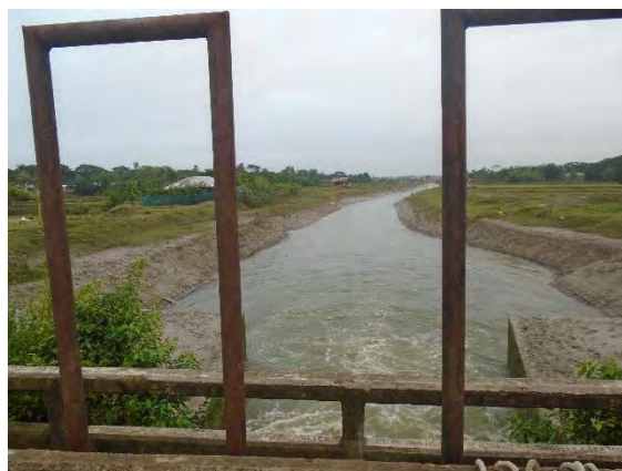
Figure: Outfall of Telikhali catchment
