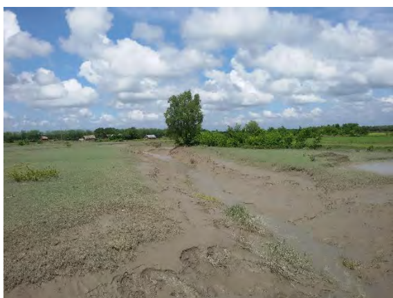
Figure: Siltrated up Offtake of Golaimari Sluice
