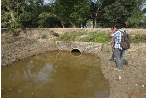
Figure 7, Culvert at the Northern section of internal drain
