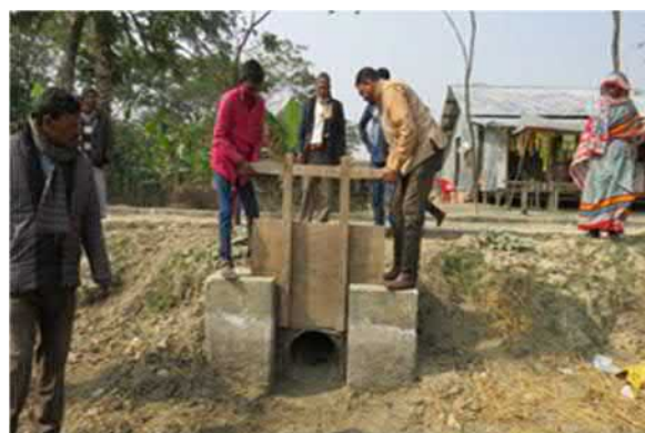
Figure 2: Construction of Box culvert in polder 43/1A
