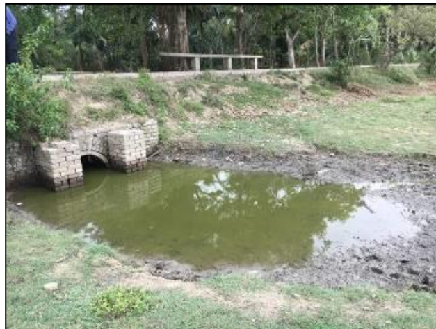
Figure 7: Second culvert connecting the internal drain with the Saduria Khal
