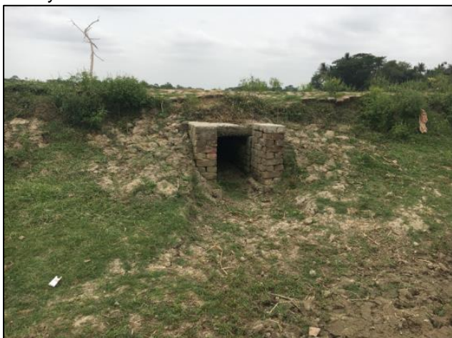
Figure 6: First culvert connecting WMU 1 and WMU 2
