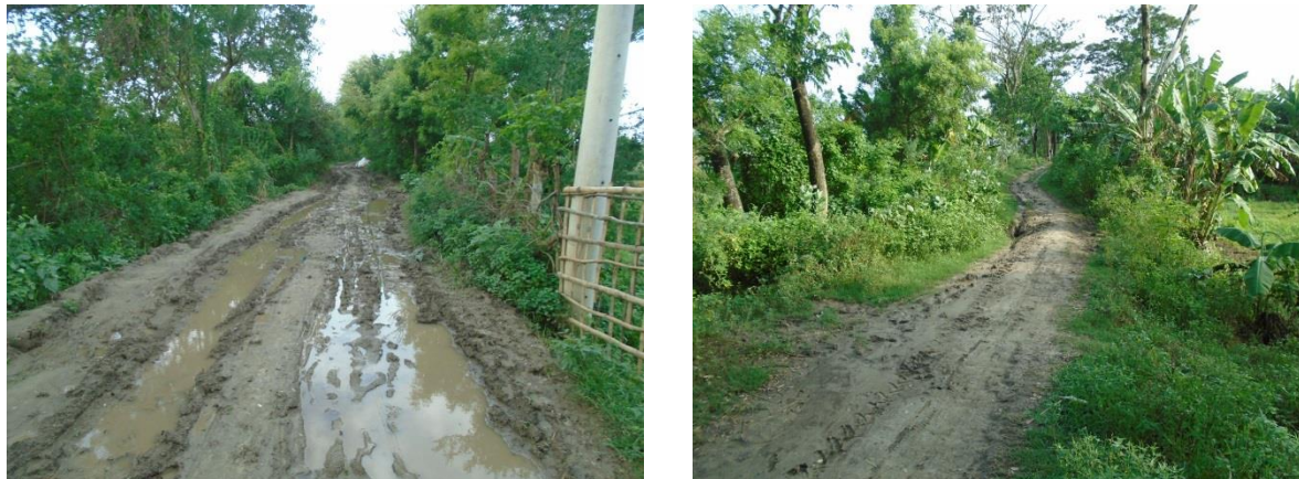
Photo 4.1 Existing Status of Embankments
