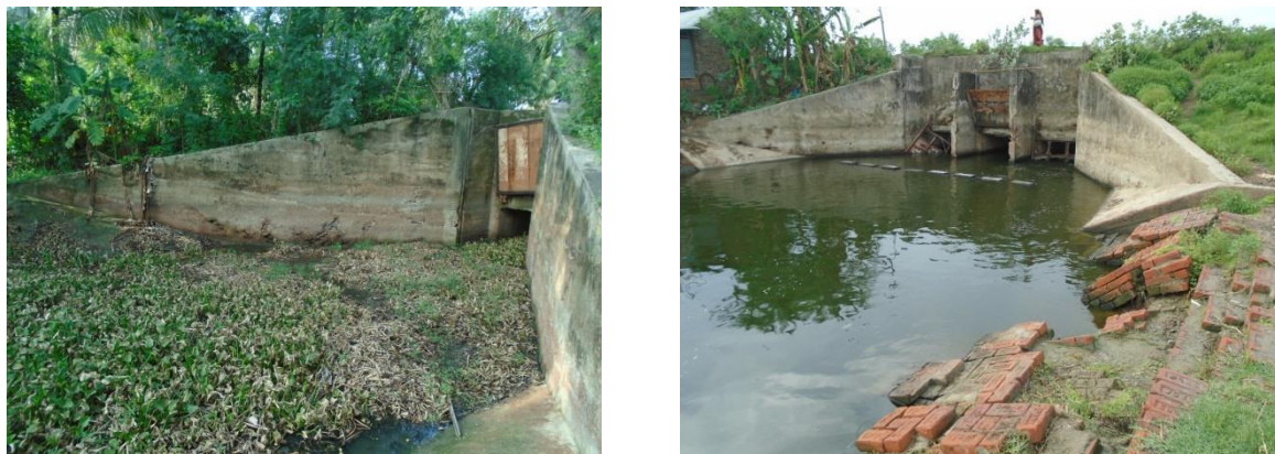
Photo 4.2 Existing Status of Kuloti Sluice and Pashkhali Sluice at Polder 28/1
