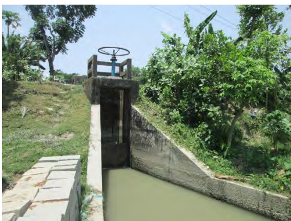
Figure: Natuar khal Sluice
