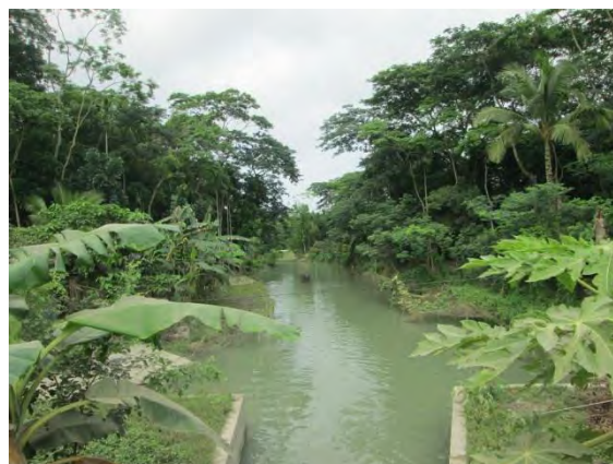
Figure: Rajabaria khal Sluice
