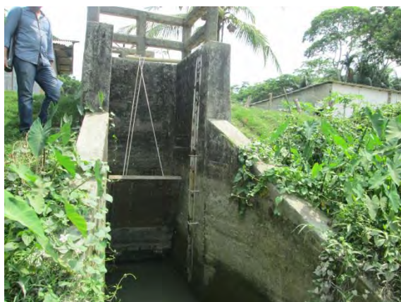
Figure: R/S of Hajikhali Sluice
