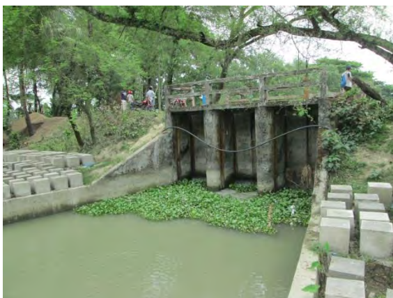
Figure: Katakhal Sluice
