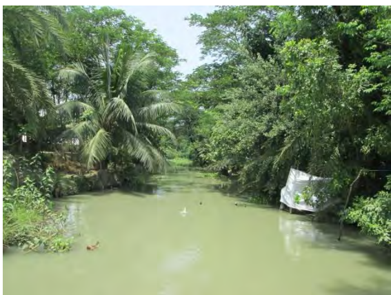
Figure: Shuddhurbari khal Sluice
