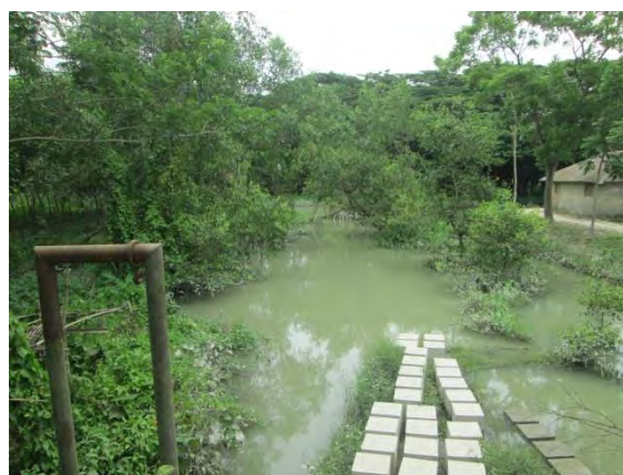
Figure: Outfall of Taltola catchment
