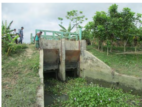
Figure: R/S of Marichbunia Sluice
