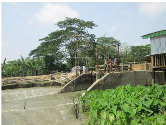
Figure: R/S of Bauria Sluice (under construction)
