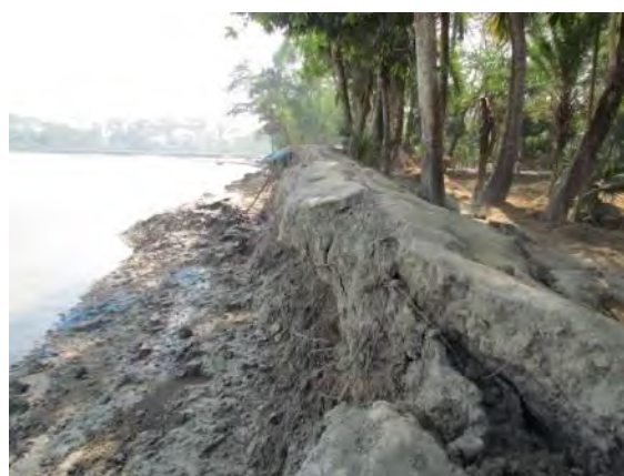
Figure: Embankment erosion at Dari Baherchar (Boloikati Village)
