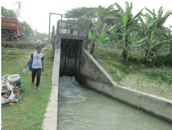
Figure: Fultola Sluice
