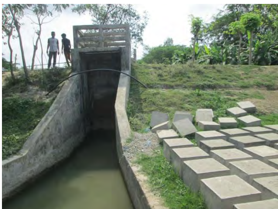
Figure: Koyer khal Sluice
