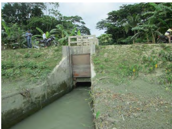
Figure: R/S of Rajabaria khal Sluice
