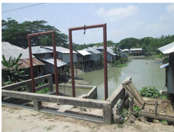
Figure: R/S of Amkhola Sluice
