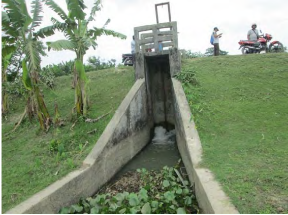
Figure: R/S of Patukhali Sluice
