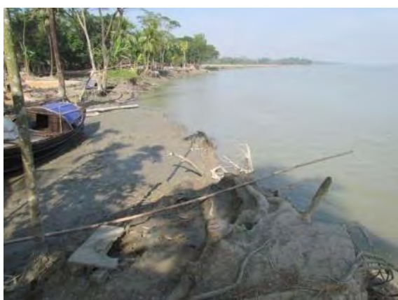
Figure: Embankment erosion at Dari Baherchar (Boloikati Village)
