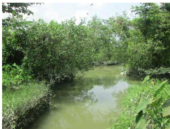
Figure: Outfall of Hajikhali catchment
